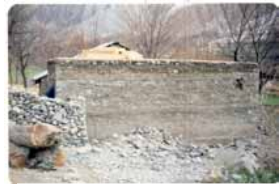
Fig.7: Newly constructed houses through technology transfer after 1991, Chitral earthquake
