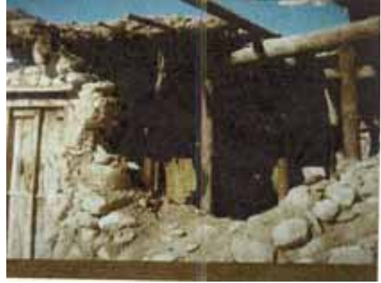
Fig. 4: Damaged village house in Chitral, 1991 earthquake
