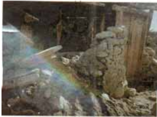
Fig.5: Destroyed village house in Chitral, 1991 earthquake
