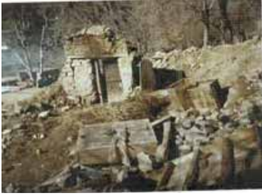
Fig.3: Destroyed village house in Chitral, 1991 earthquake
