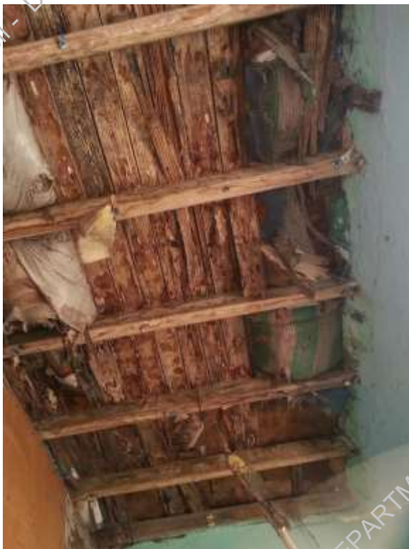
Plate-9: Bad condition wooden flooring
