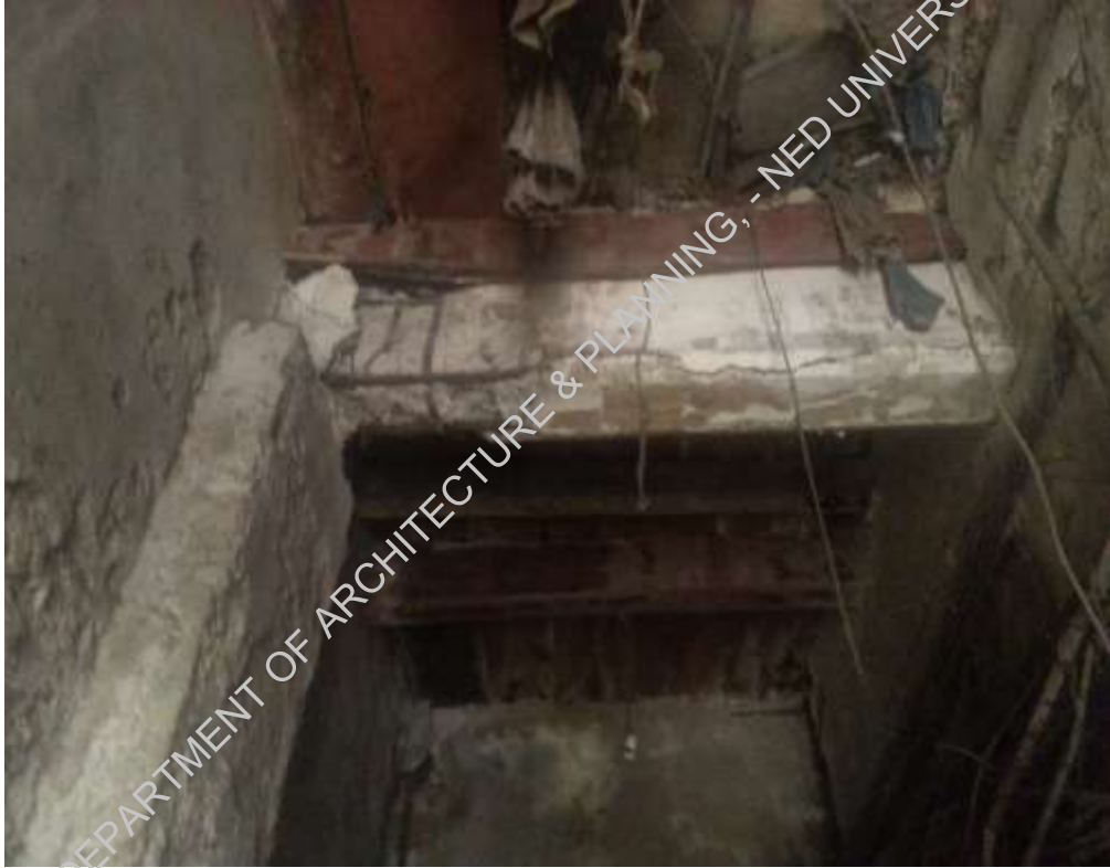
Plate-7: Bad condition of slab due to punctures and seepage from plumbing lines
