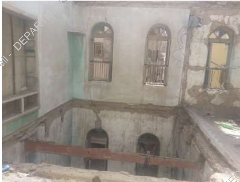
Plate-10: collapsed slab at 3 rd floor
