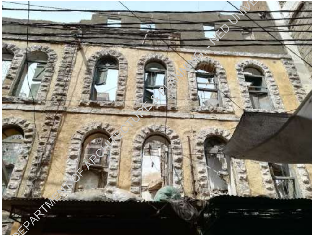
Plate-6: Loose stone masonry is visible
