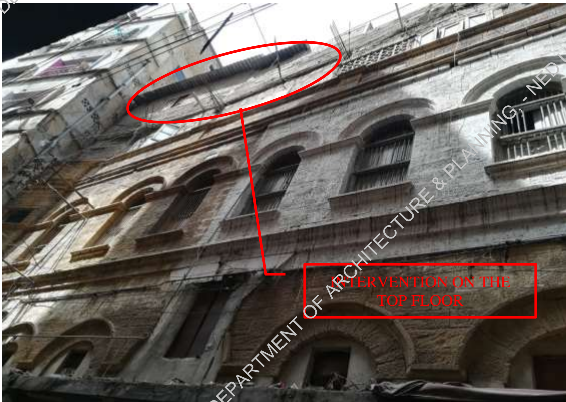
Plate-1: Front Façade- loose stone masonry can be noted at few places. Additional floor on top is also visible
