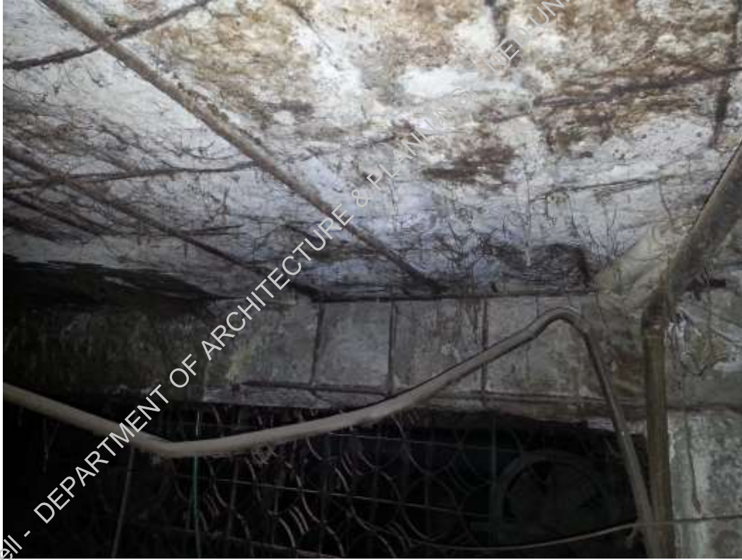
Plate-5: Concrete construction done later on, in bad condition, concrete cover has fallen off.
