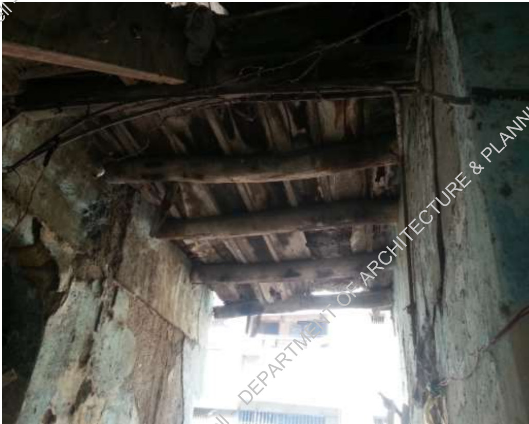
Plate-10: Bad condition of original timber flooring and walls at ground floor
