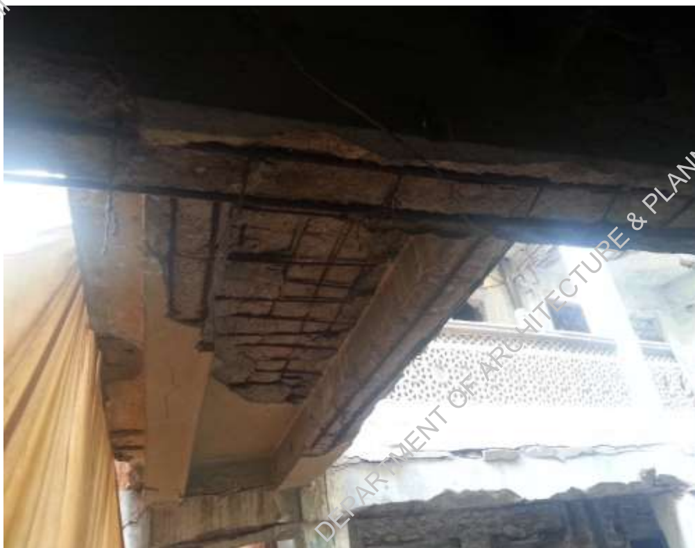
Plate-7: concrete cover fallen off
