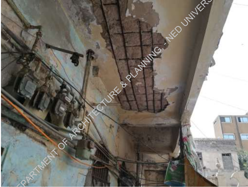
Plate-8: reinforced concrete slab in bad condition, concrete cover has fallen off.
