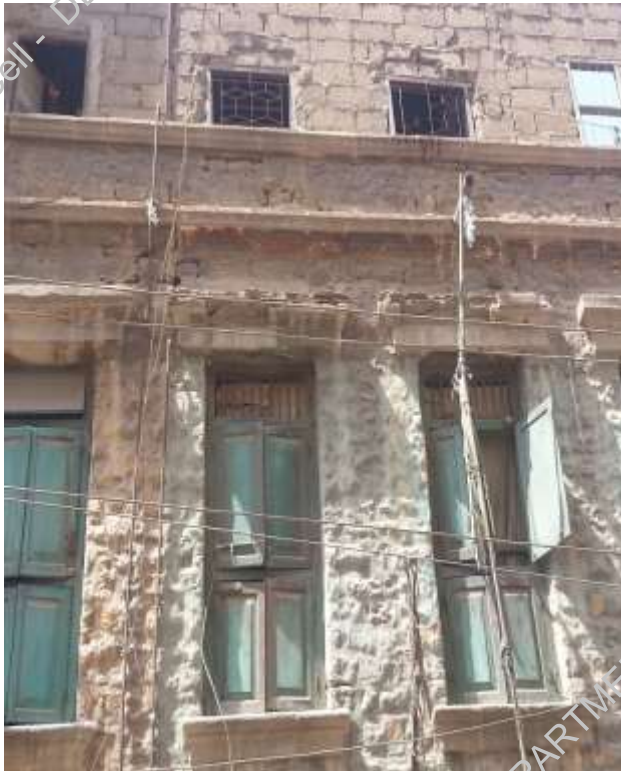
Plate-2: bad condition of masonry in façade
