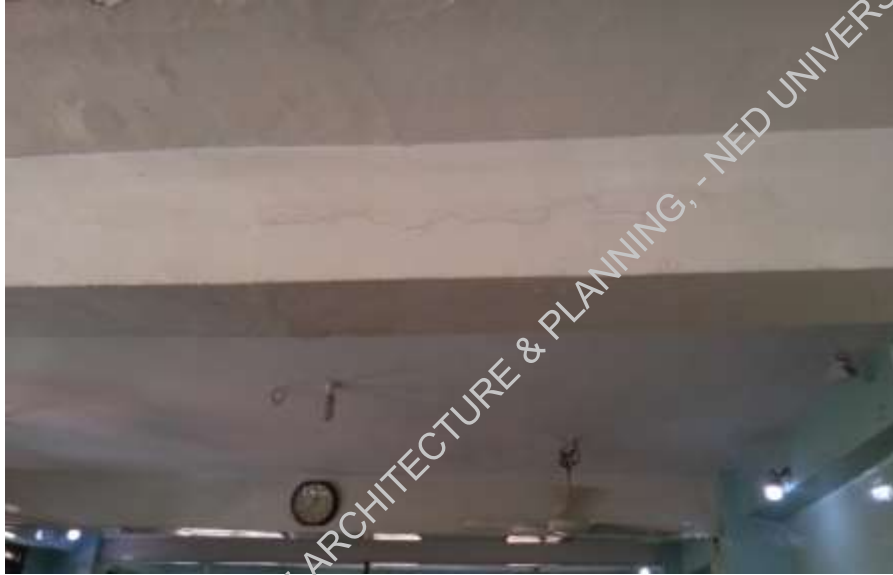
Plate-5: horizontal cracks in roof beams
