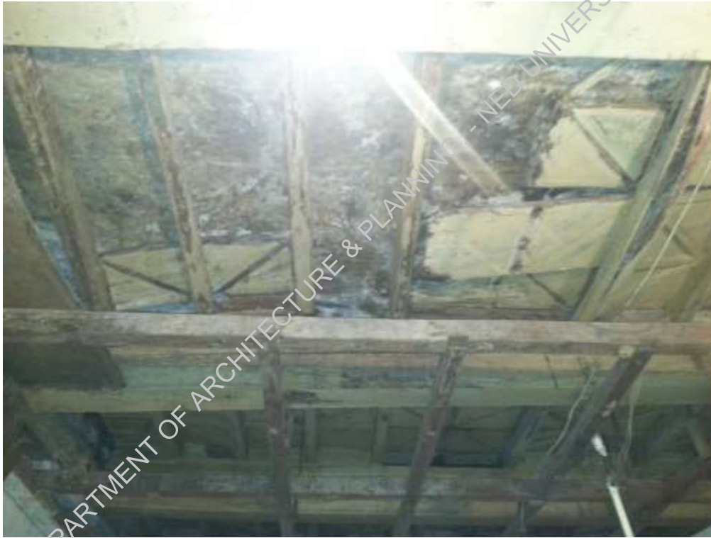
Plate-8: wooden deck condition inside
