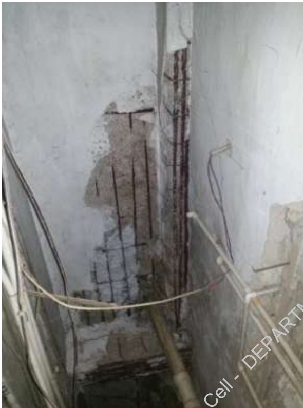
Plate-5: concrete cover damage
