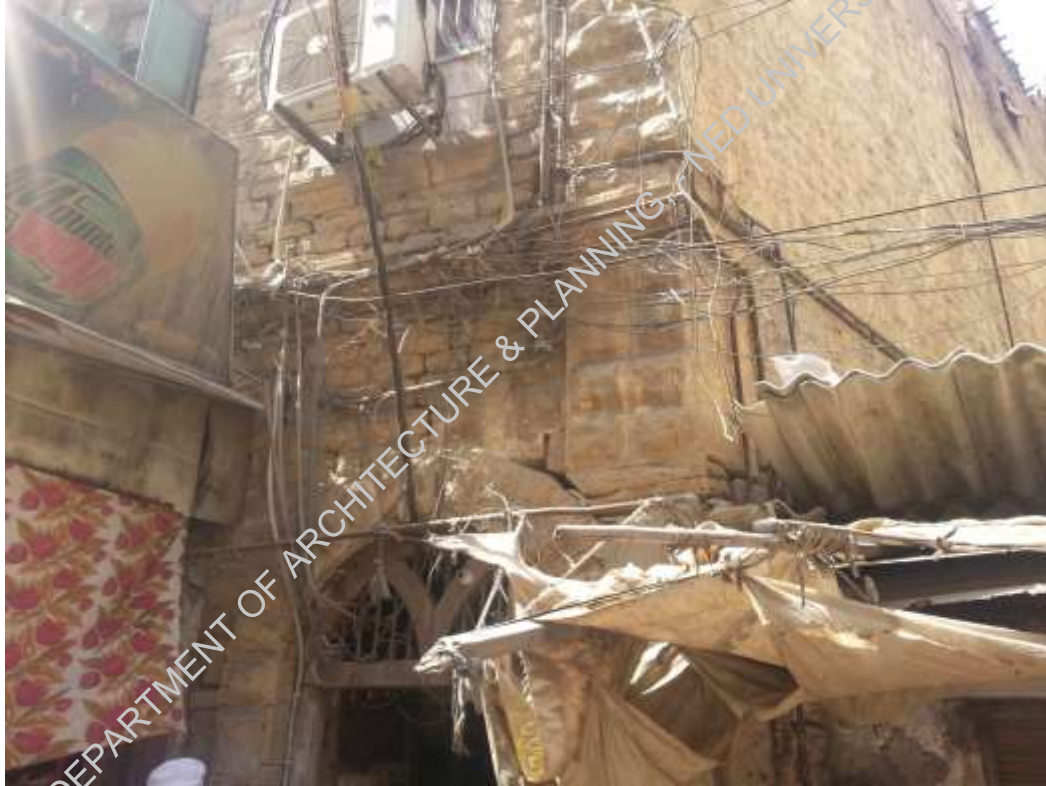
Plate-4: vertical cracks observed
