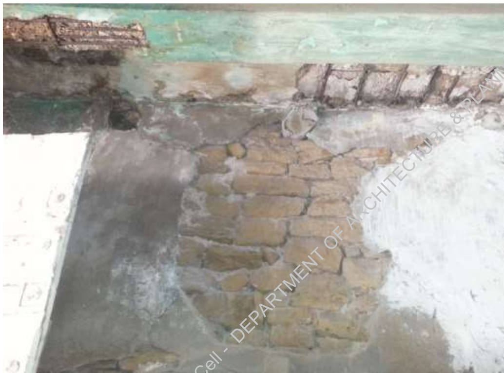
Plate-6: Loose stone masonry is visible
