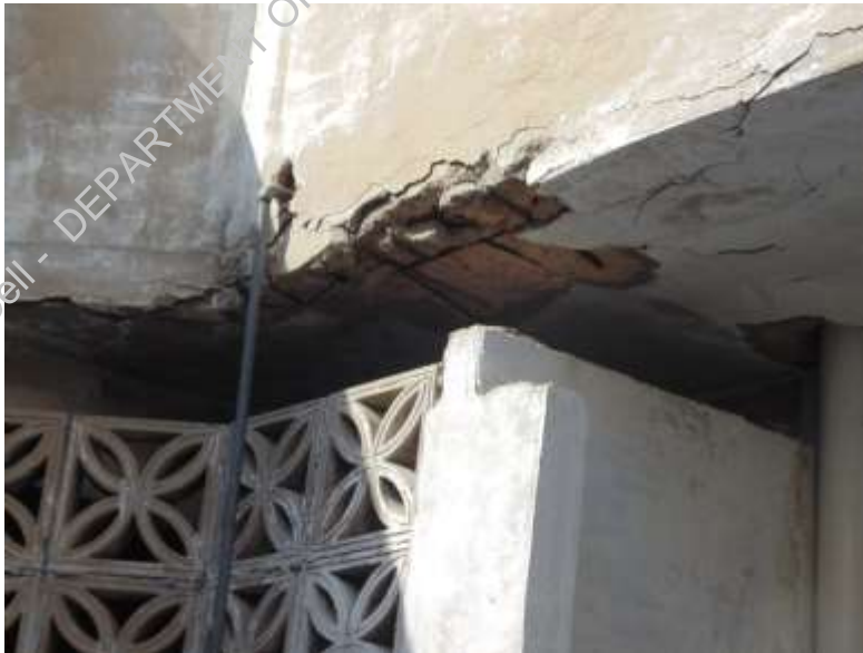
Plate-6: Concrete cover damage
