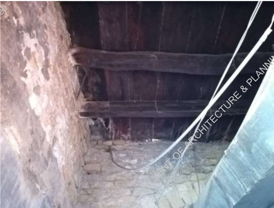
Plate-5: Bad condition of original timber flooring and walls at ground floor
