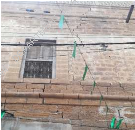
Plate-5: vertical cracks on both floors in façade
