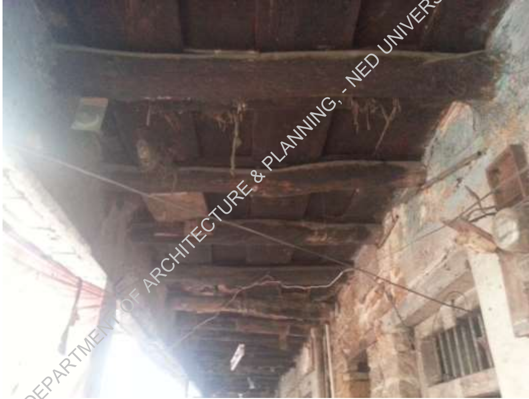
Plate-4: original deck in bad condition,
