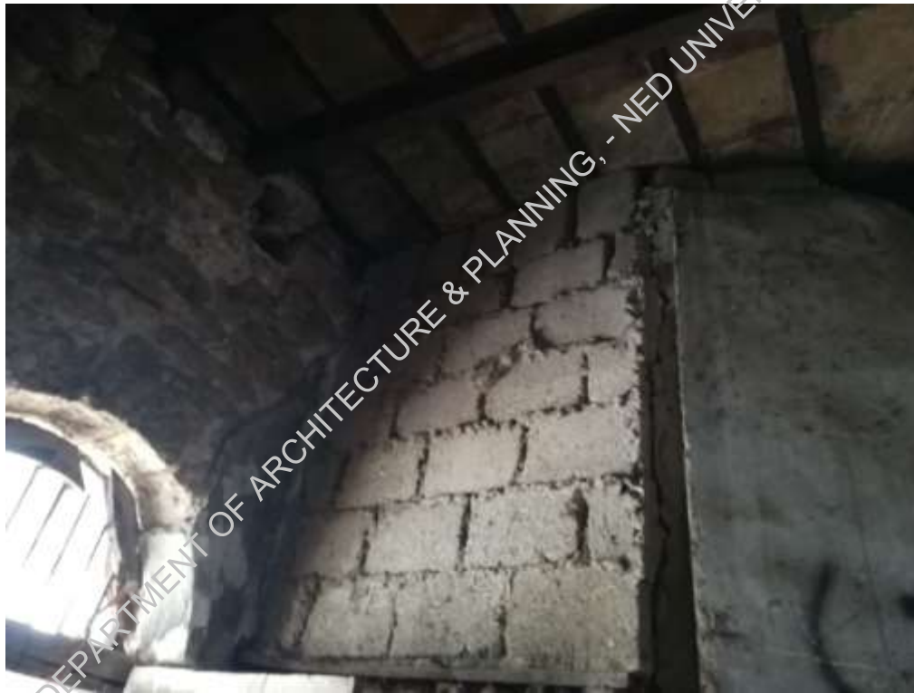
Plate-6: Loose stone masonry is visible
