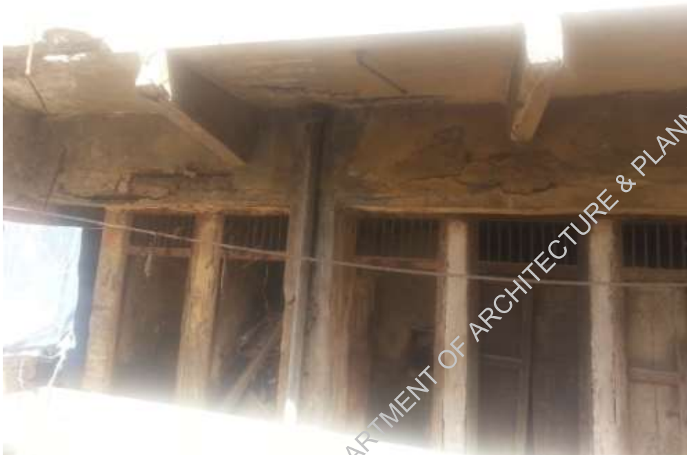
Plate-9: cracks observed above lintel
