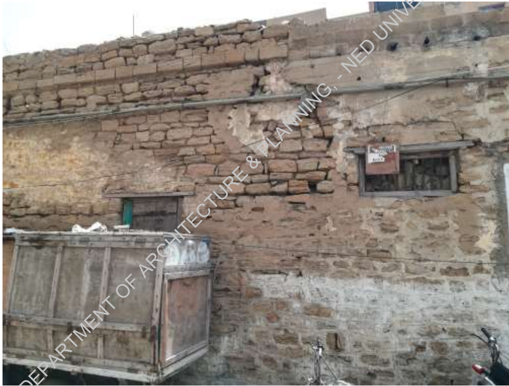
Plate-6: Loose stone masonry is visible
