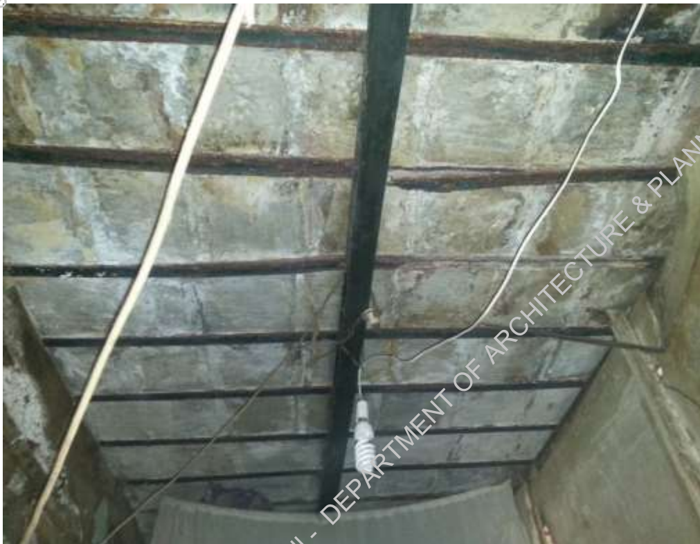
Plate-7: Bad condition of roof slab due to punctures and seepage from plumbing lines
