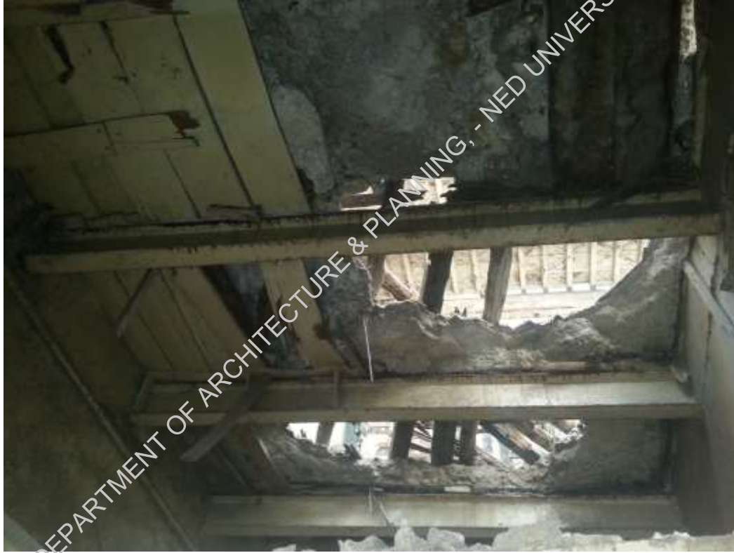
Plate-4: slab collapsed
