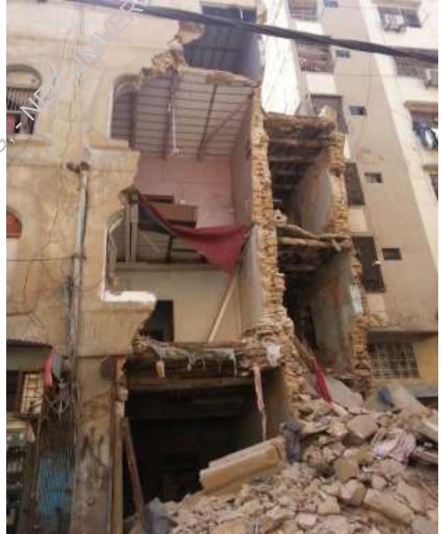
Plate-3: After collapse of rear side
