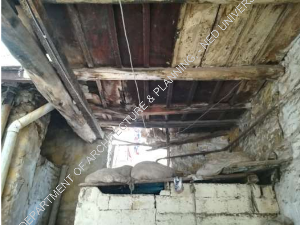
Plate-4: Bad condition of original timber flooring and walls
