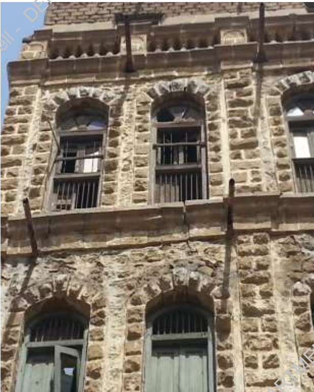
Plate-2: Wide cracks at the façade of building
