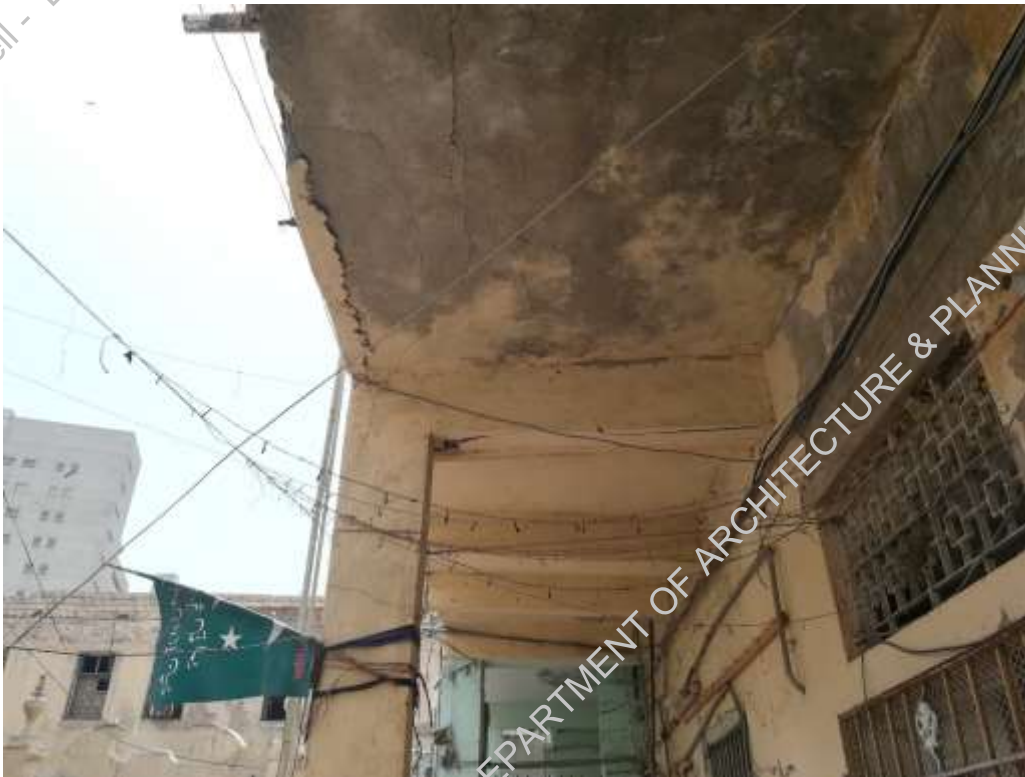
Plate-7: Bad condition of reinforced concrete construction of central court
