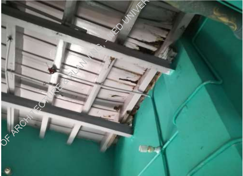
Plate-6: Deformed timber slab resting on MS beams installed at later stage.
