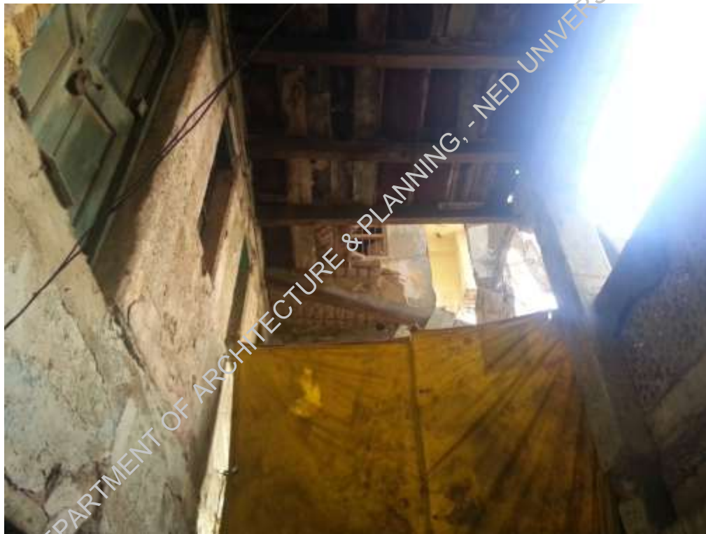
Plate-6: bad condition of timber slab
