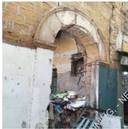
Plate-6: Cracks around the arch
