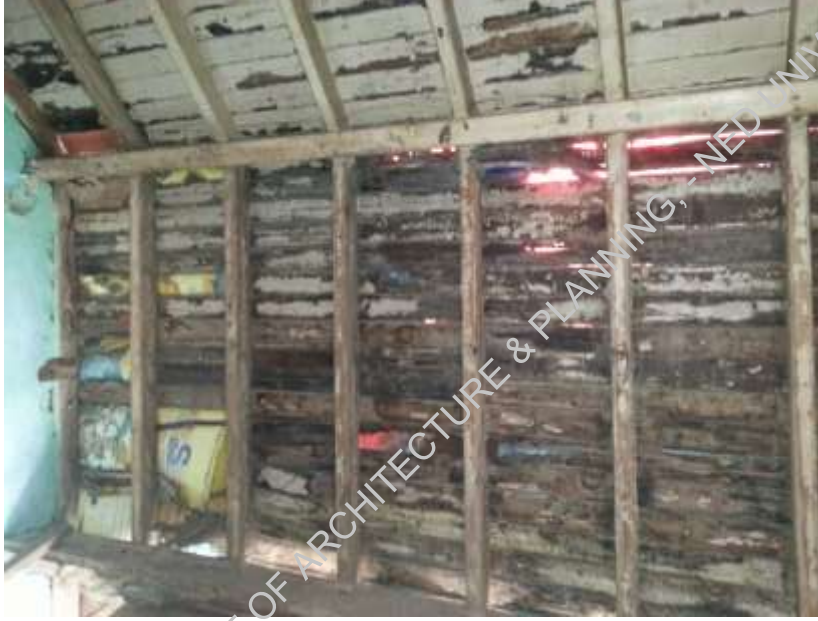
Plate-10: Bad condition of original timber flooring
