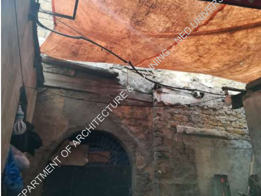
Plate-10: Loose masonry visible
