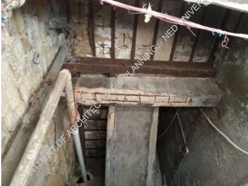
Plate-4: reinforced concrete slab in bad condition, concrete cover has fallen off. It has be strengthened still in very bad condition
