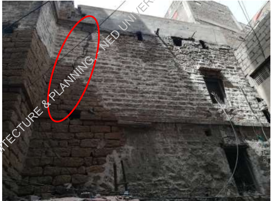
Plate-2: Wide cracks at the rear façade of building
