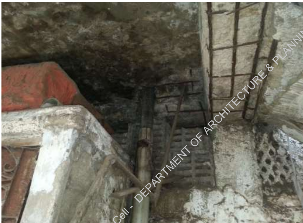
Plate-6: Exposed rebar's subject to rusting
