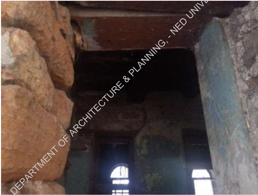
Plate-10: Bad condition of original timber slab
