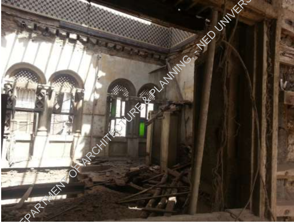
Plate-10: slab collapsed
