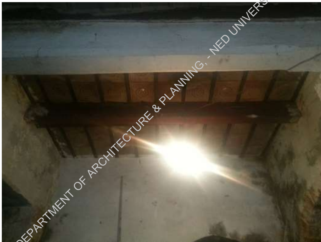
Plate-5: Original timber beam intact
