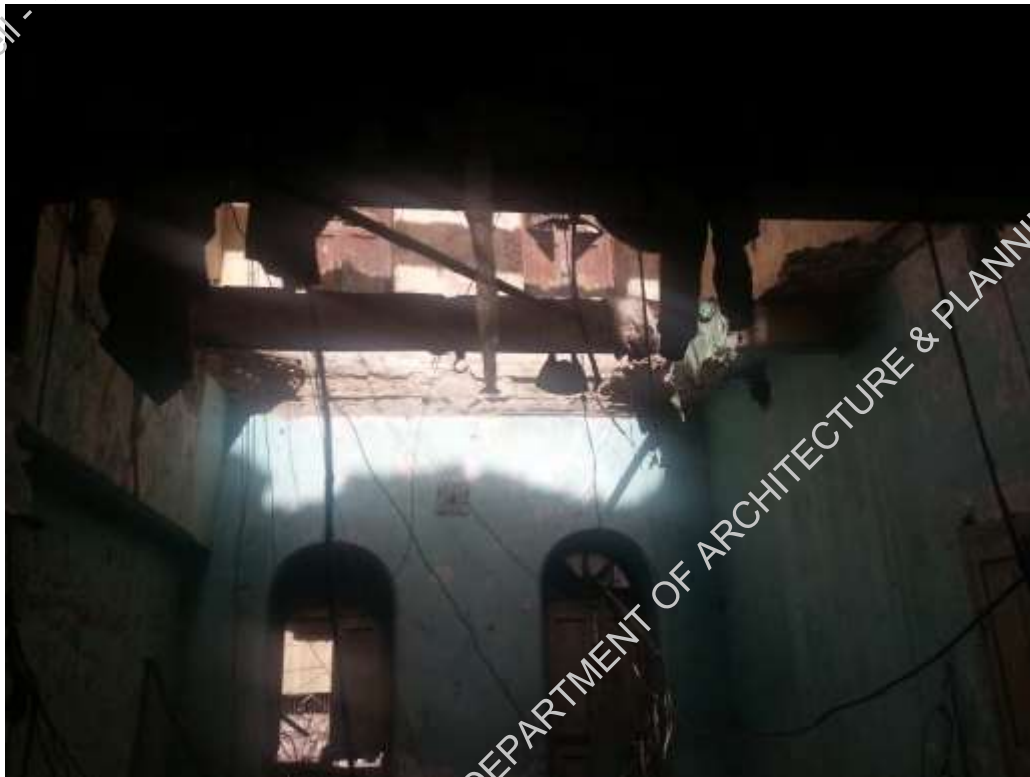
Plate-10: collapsed slab at 2 nd floor
