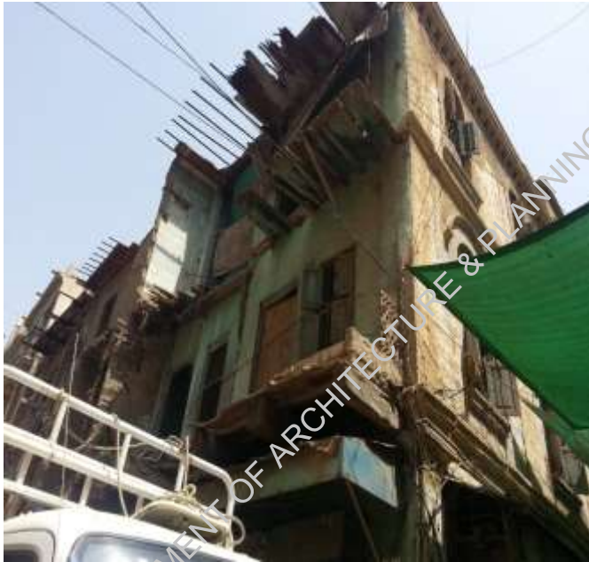
Plate-2: original wooden structural elements in deteriorated condition
