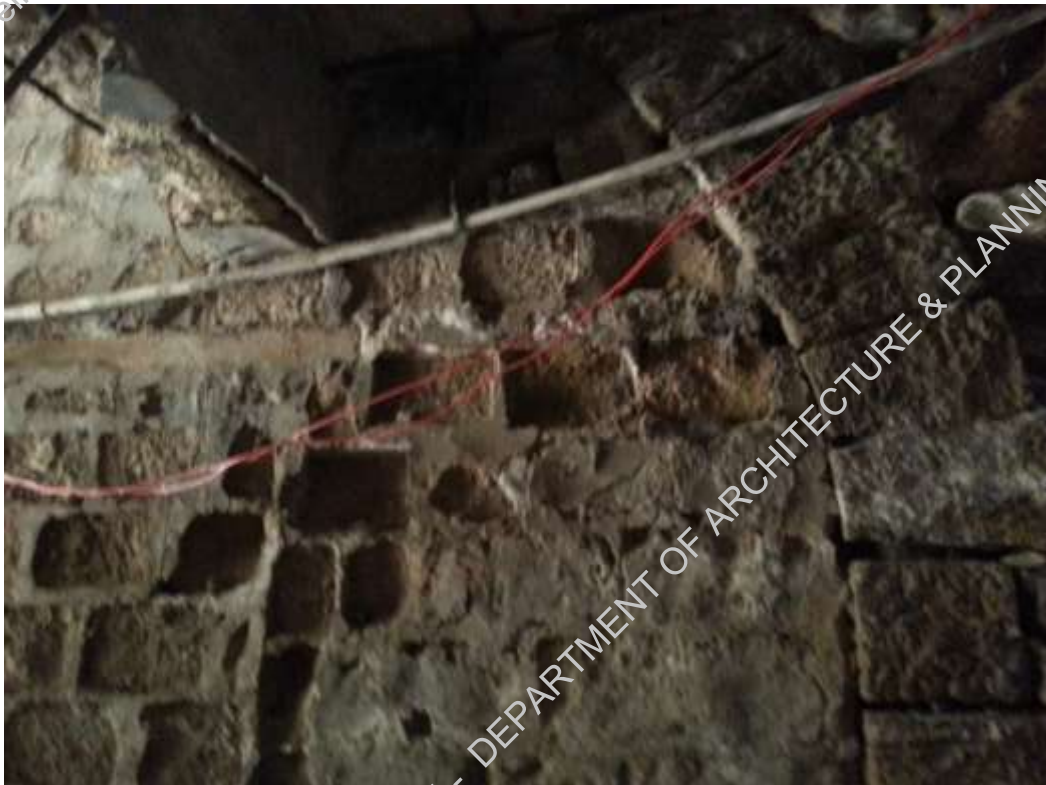
Plate-5: deteriorated stone and mortar
