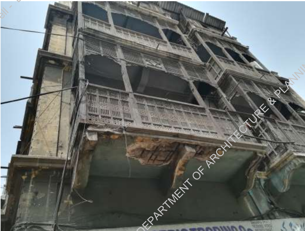
Plate-5: plaster fallen off due to lack of maintenance
