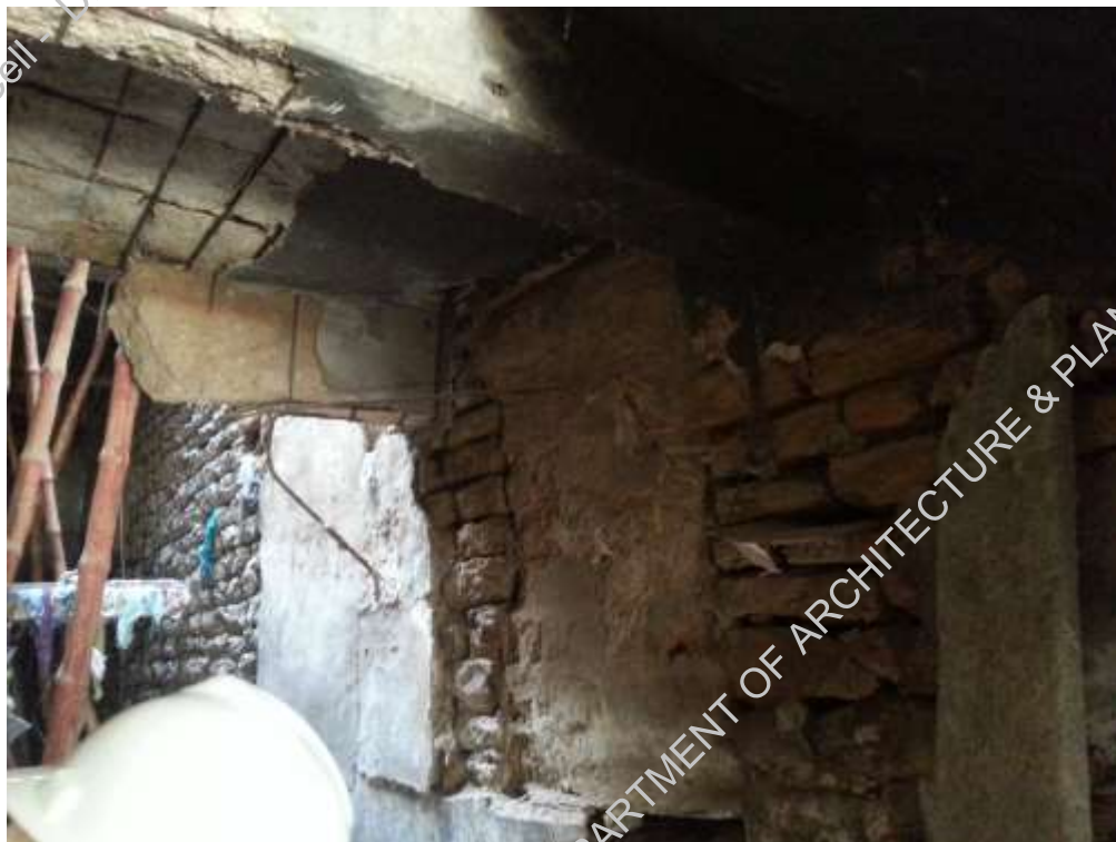
Plate-9: opening in stone walls needs to be filled
