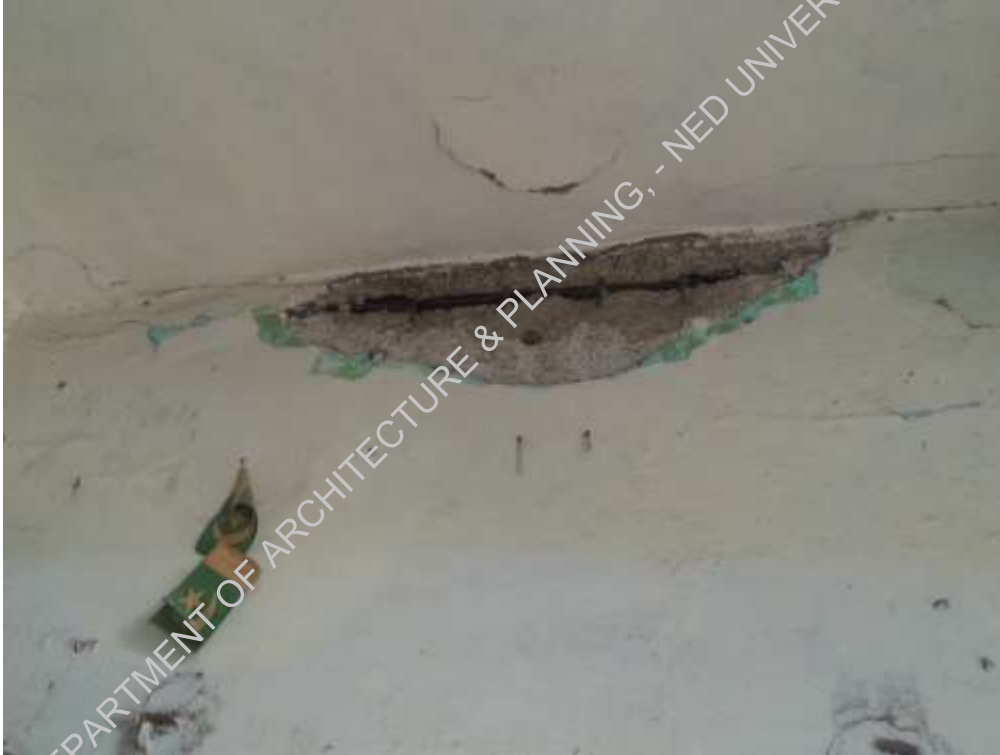
Plate-8: damage due to seepage
