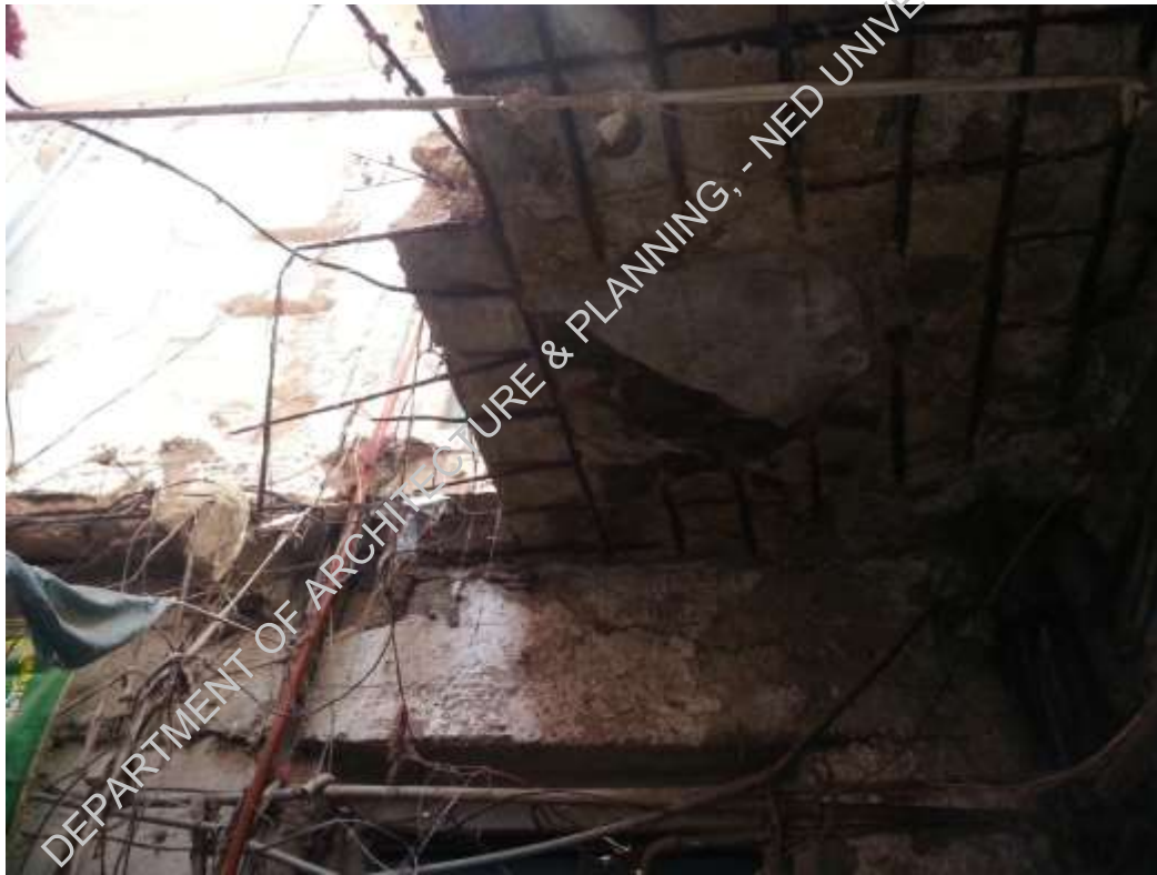
Plate-7: Bad condition of roof slab due to seepage from plumbing lines
