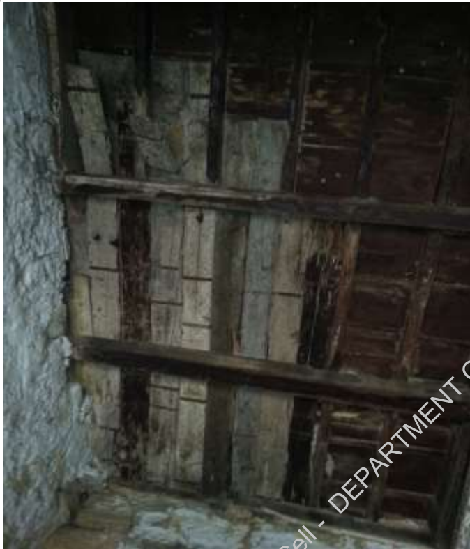
Plate-4: Timber slab in bad condition
