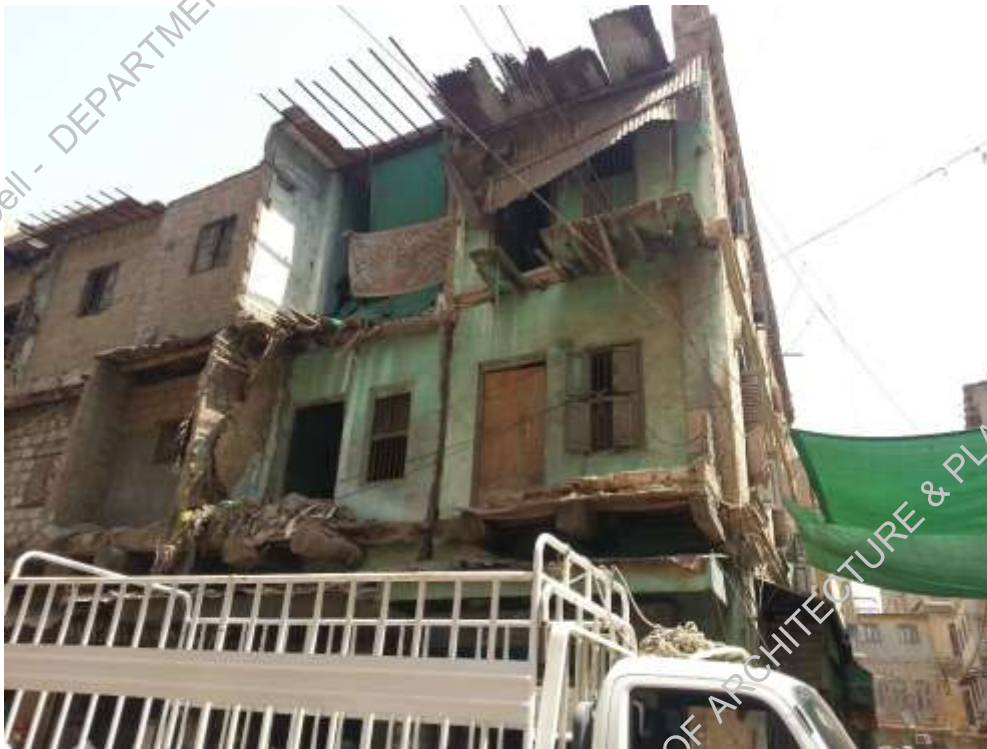
Plate-1: side Façade- Partially Collapsed
