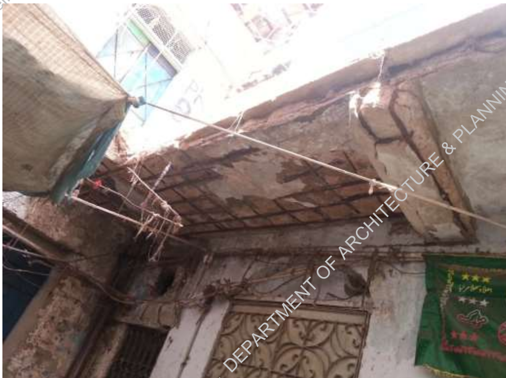
Plate-8: Projection plaster being fallen off
