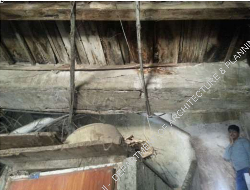
Plate-5: Concrete construction beam deflecting
