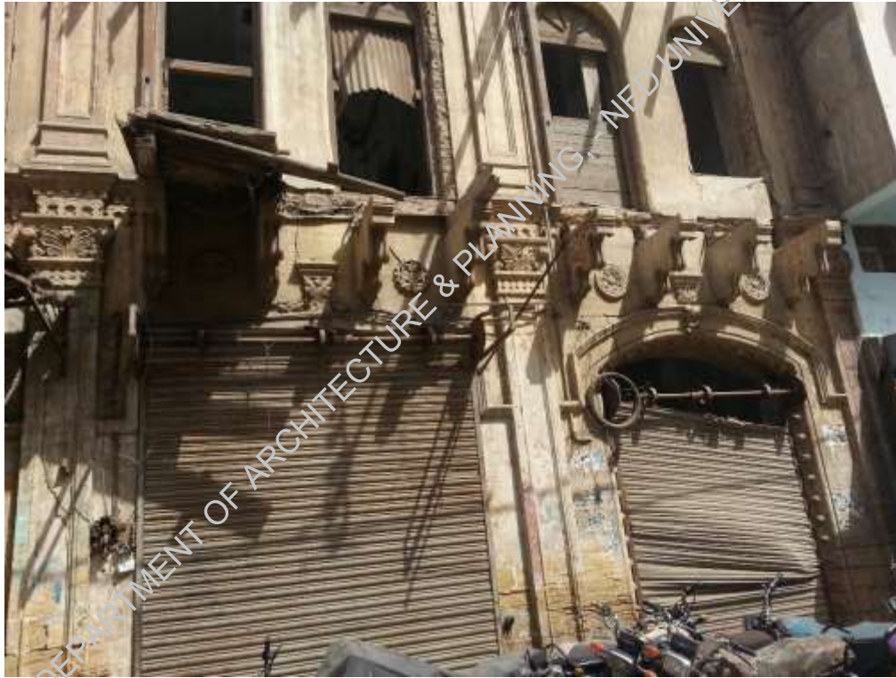
Plate-6: broken projections
