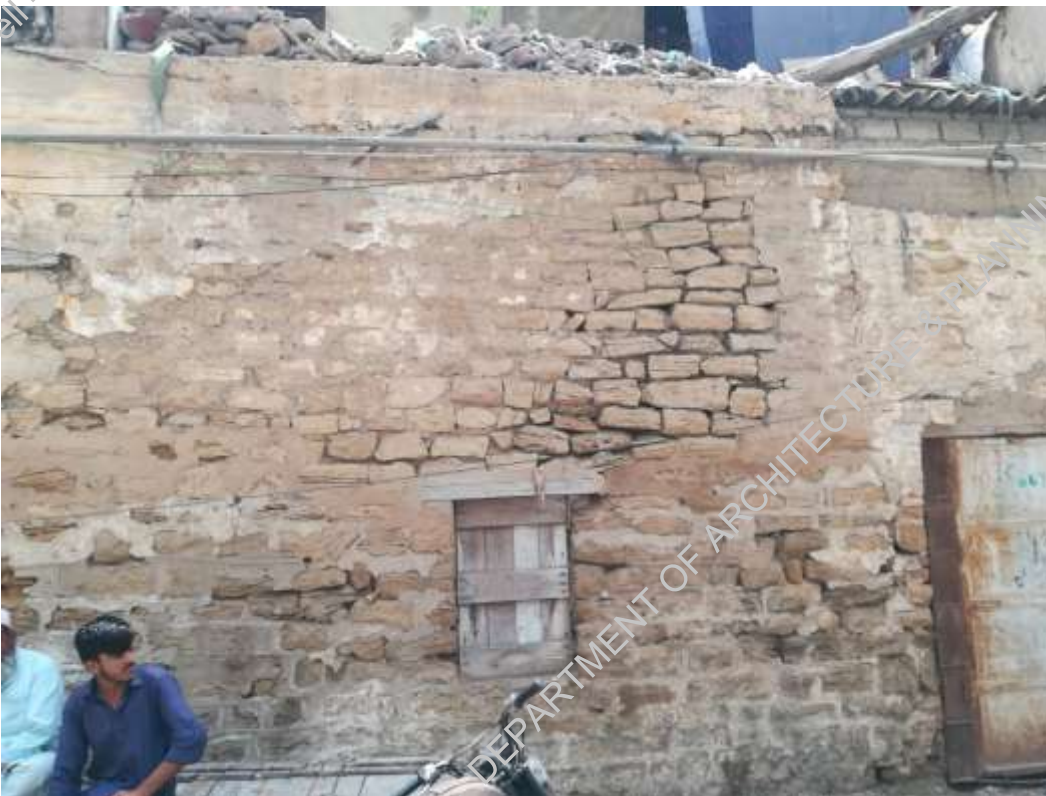
Plate-5: Loose stone masonry is visible
