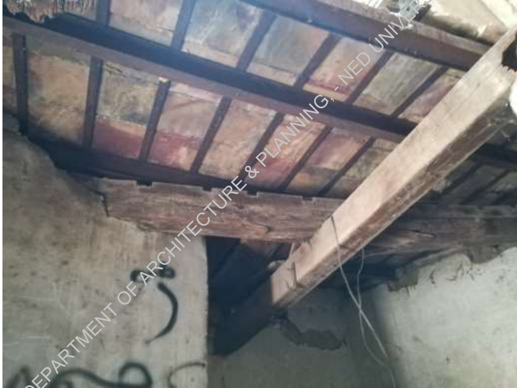
Plate-4: timber slab in bad condition,
