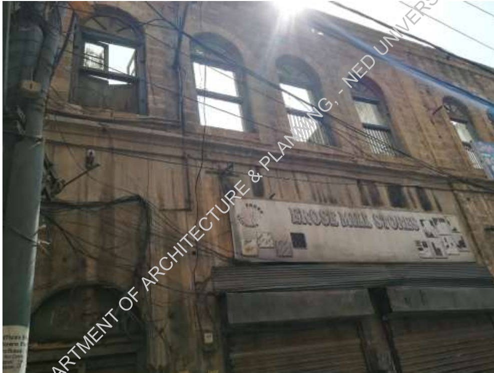
Plate-1: Front Façade- loose stone masonry can be noted at many places.
