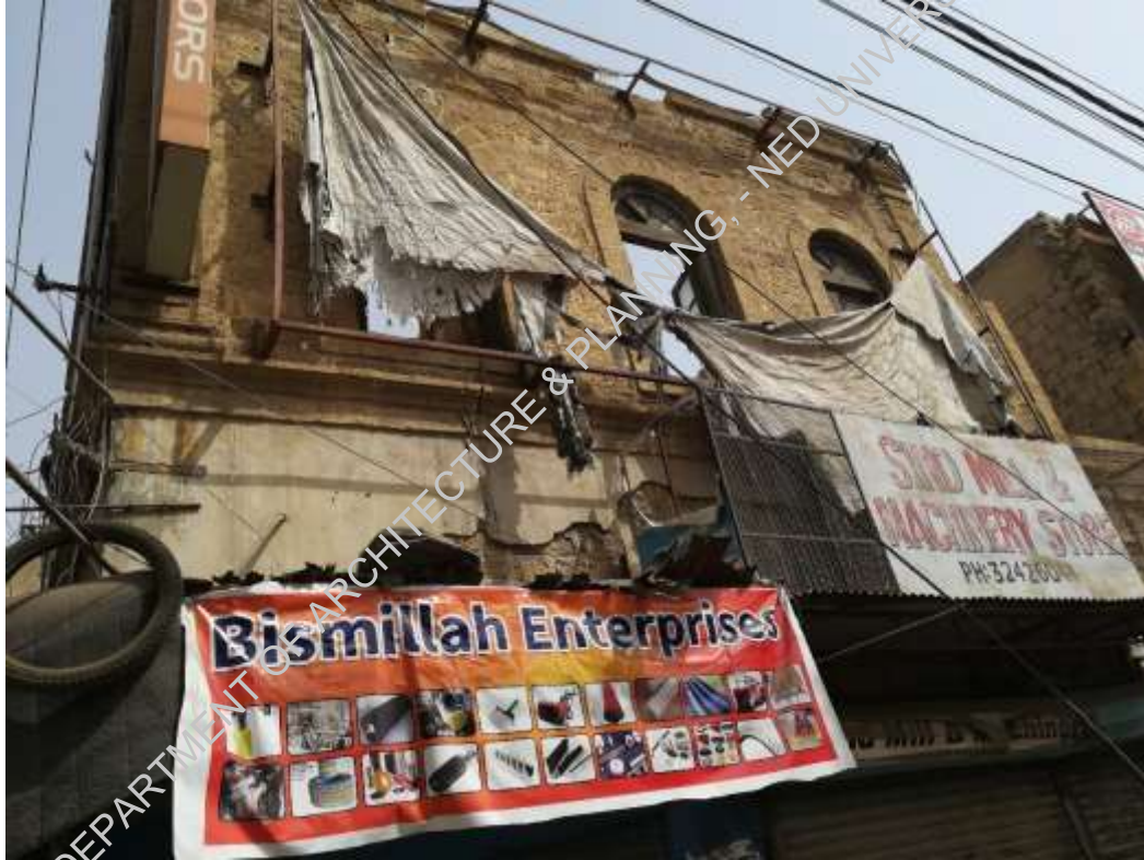
Plate-4: masonry wall is damaged due to intervention of structural steel for bill board
