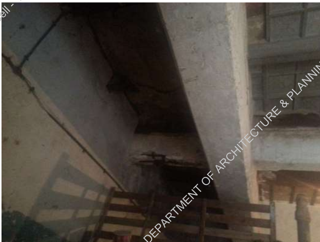
Plate-6: Concrete cover fallen off at places
