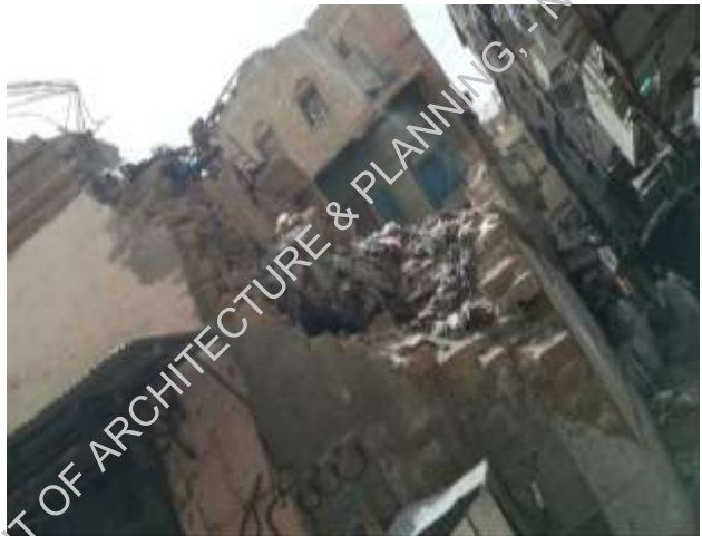
Plate-2& 3: side façade of the building collapsed
