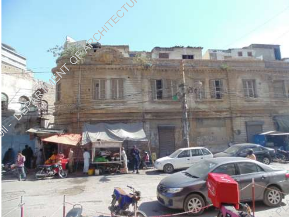
Plate-1: Front Façade- loose stone masonry can be noted at many places. Additional floor on top is also visible
