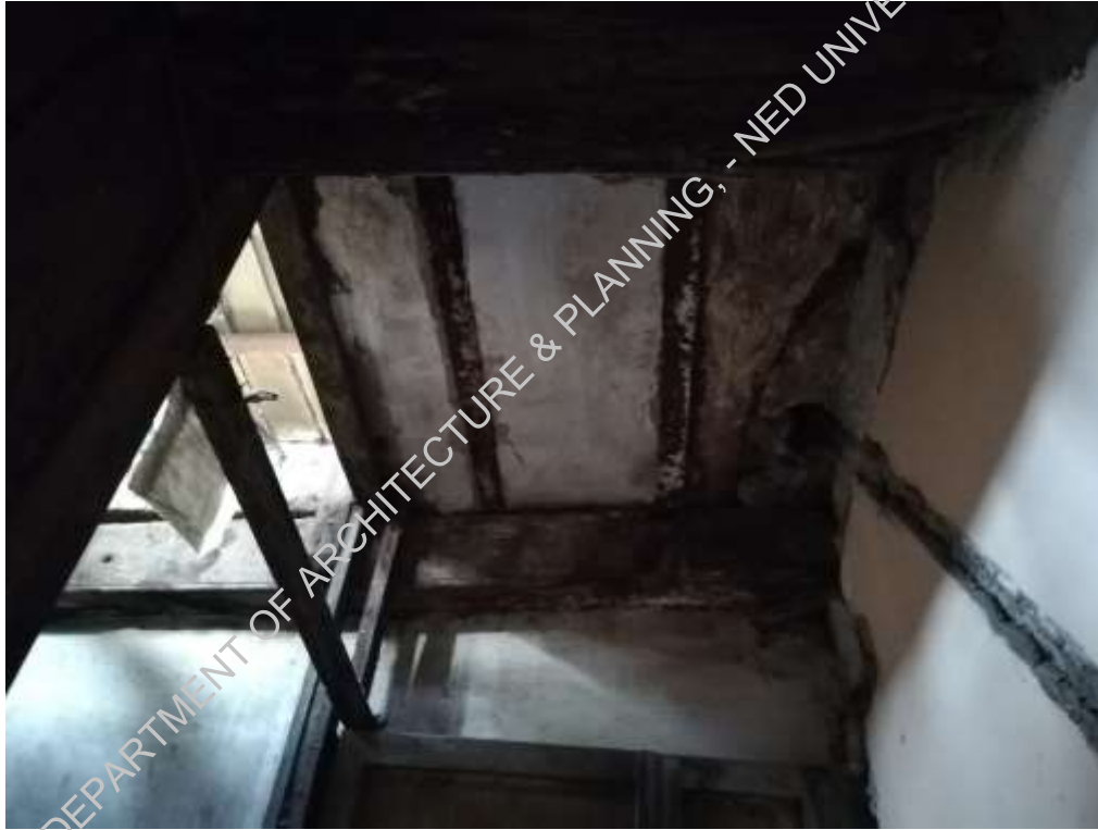
Plate-6: slab damage due to seepage
