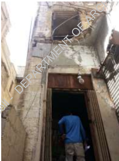
Plate-10: Bad condition of original timber flooring and walls at ground floor
