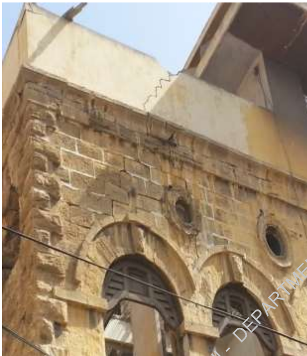
Plate-2: Wide cracks at the façade of building
