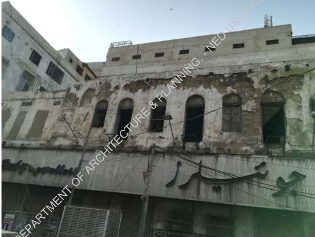
Plate-4: reinforced concrete slab in bad condition, concrete cover has fallen off. Plaster been weathered.
