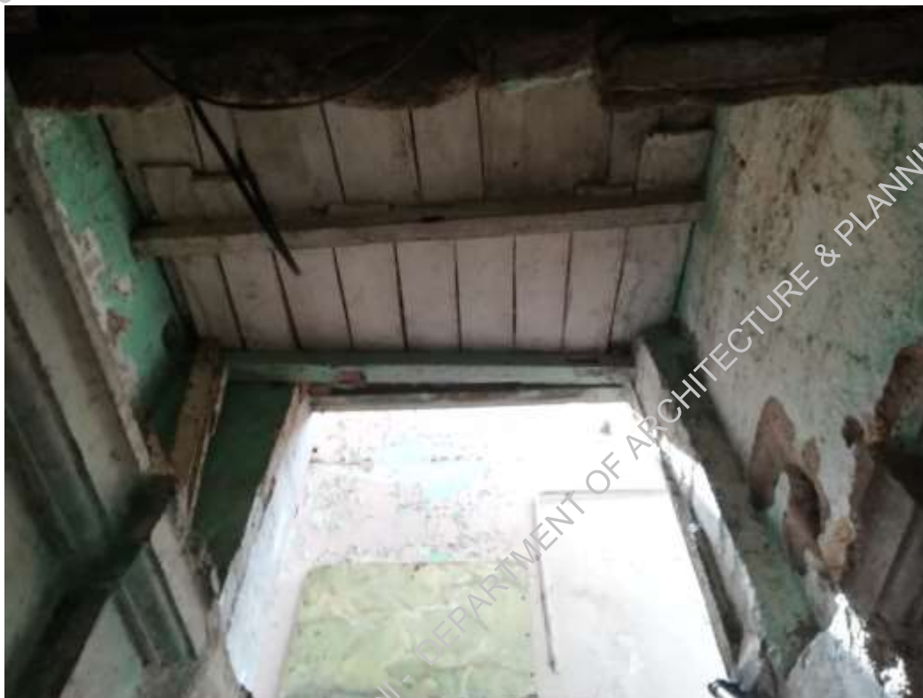
Plate-7: Bad condition of roof slab due to punctures and seepage from plumbing lines
