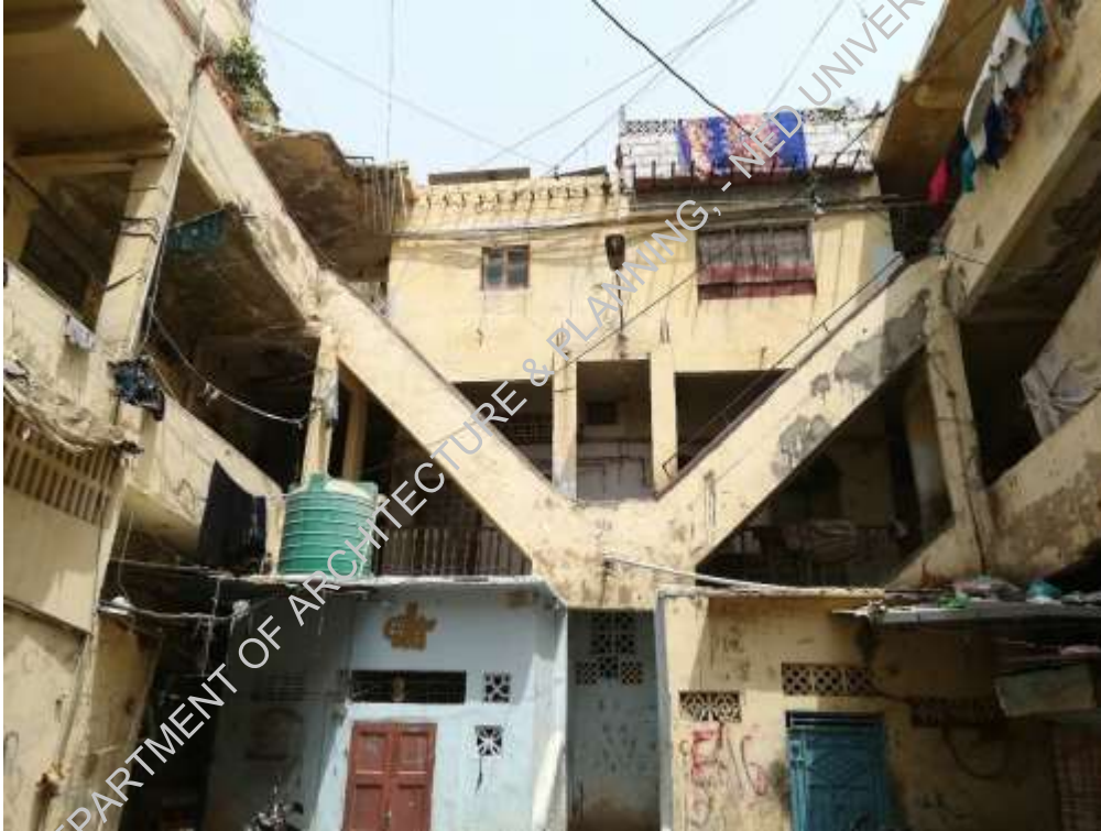
Plate-6: Central court being turned into RCC construction
