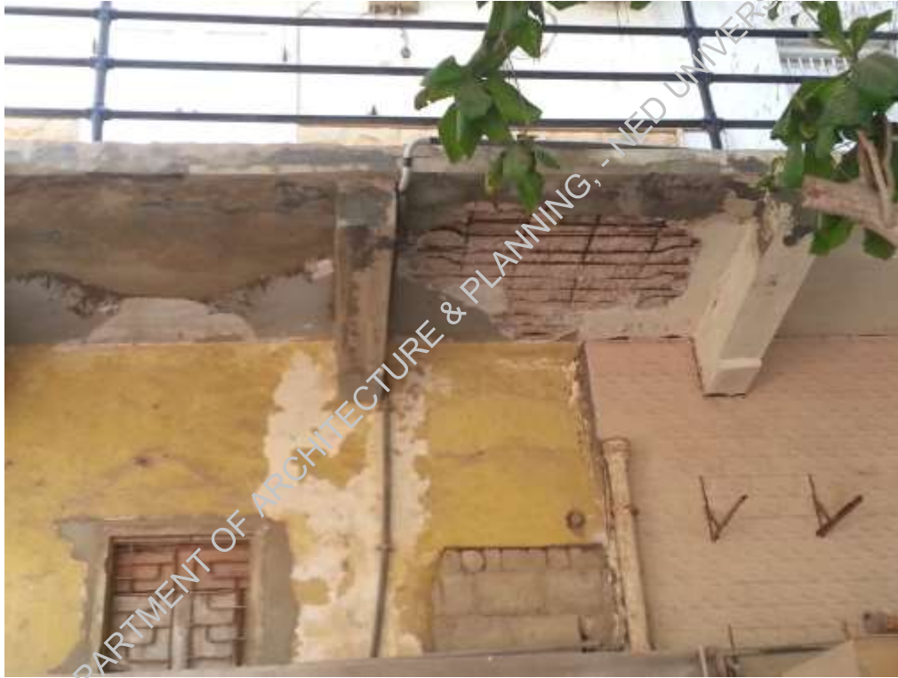
Plate-8: Concrete cover fallen off
