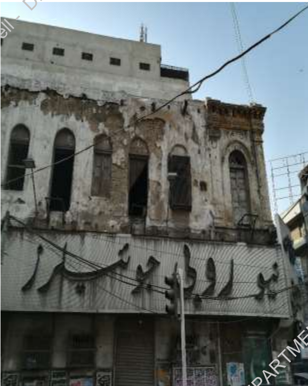
Plate-2 Plaster fallen off from the façade of building
