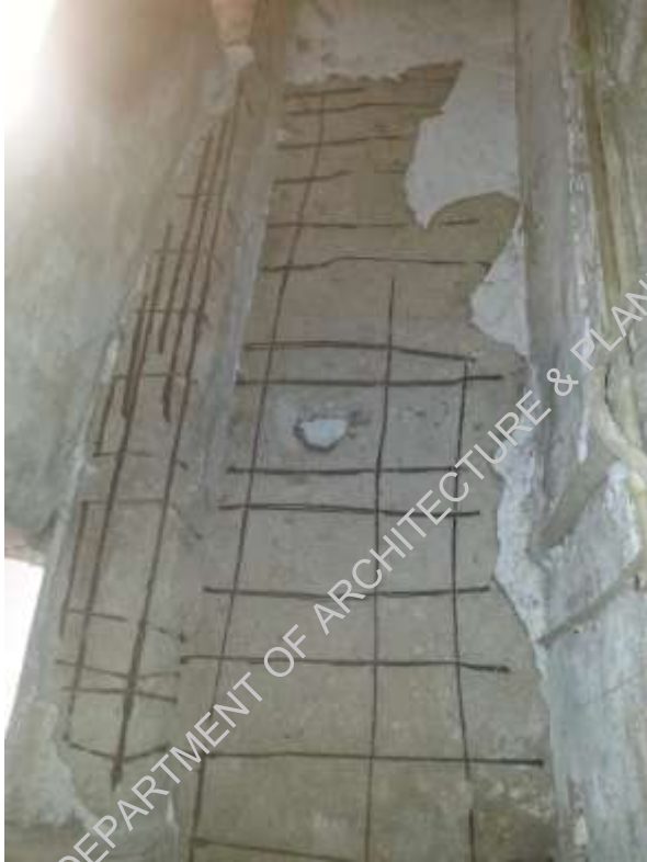
Plate-4: reinforced concrete slab in bad condition, concrete cover has fallen off.
