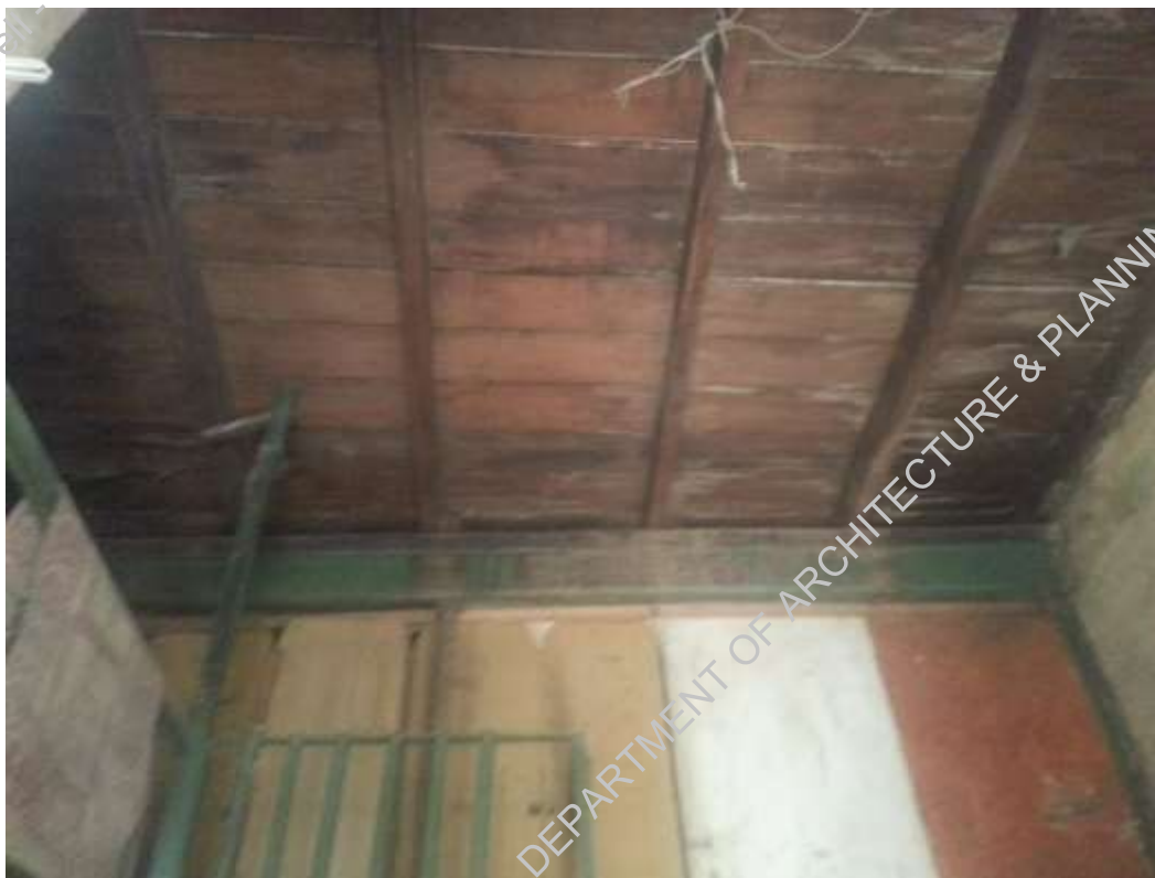
Plate-5: condition of wooden slab at ground floor
