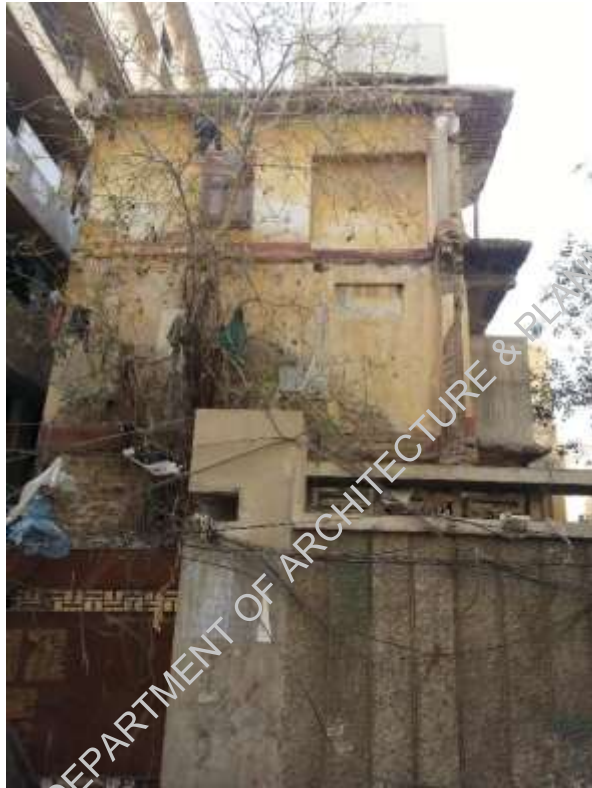
Plate-4: tree out grown from the wall tearing the wall apart
