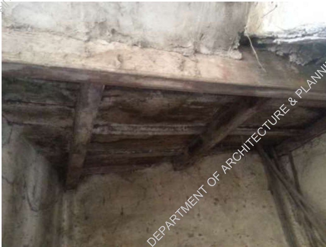
Plate-7: Bad condition of timber slab due seepage from.
