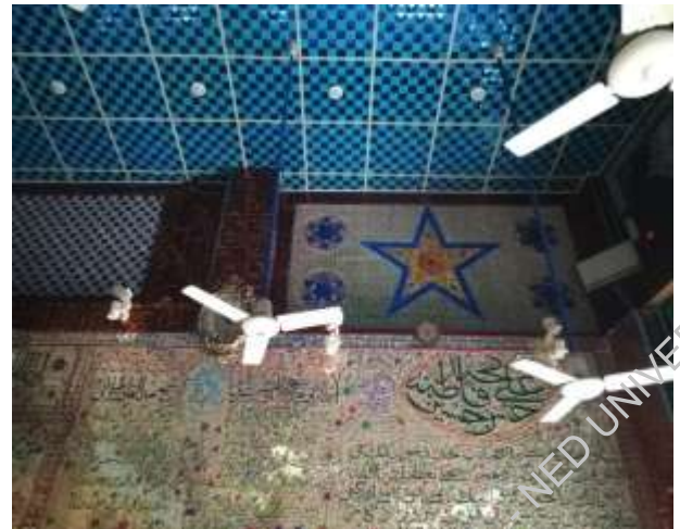
Plate-6: Walls and Columns completely covered with tiles and false ceiling hides the temporary roof laying above
