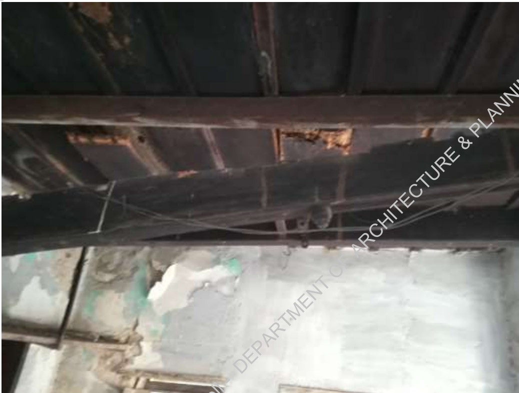
Plate-7: Bad condition of timber deck
