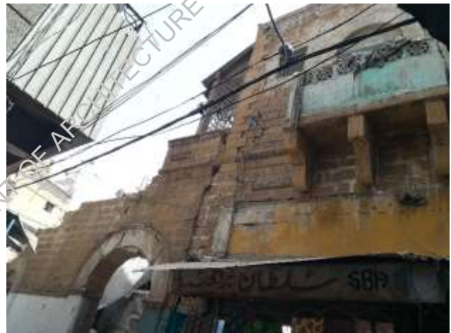
Plate-8: Cracks at location of collapse
