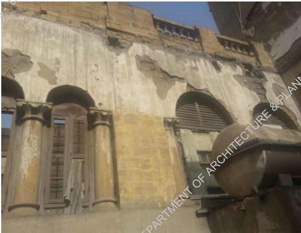
Plate-9: Bad condition of plaster and masonry at first floor
