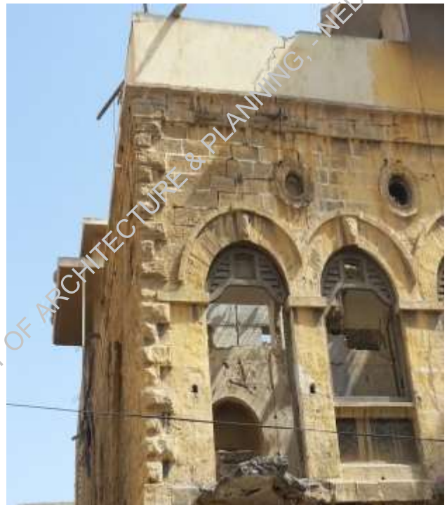
Plate-3: walls seems bulging
