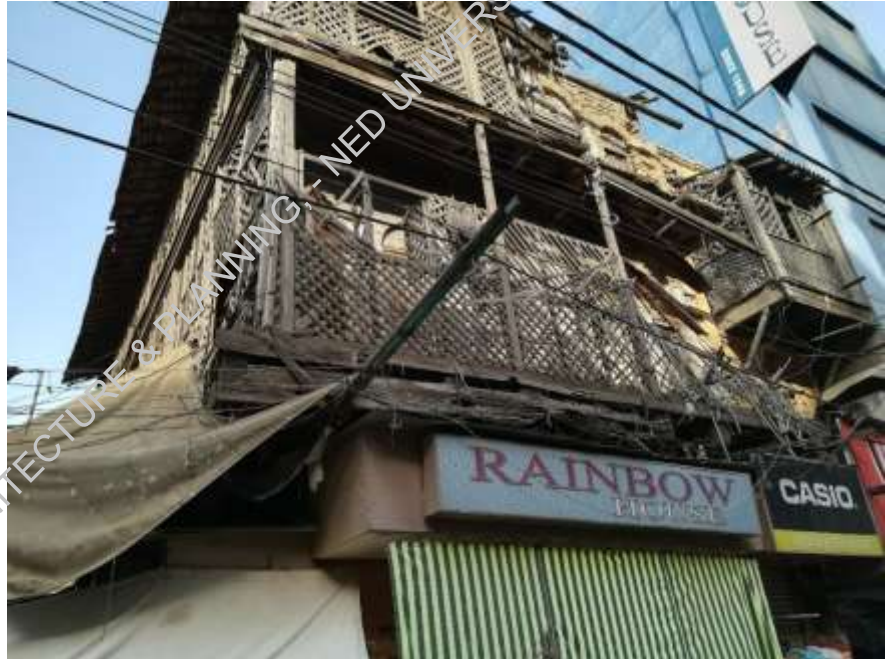
Plate-1: Front Façade- wooden jali work in bad condition.
