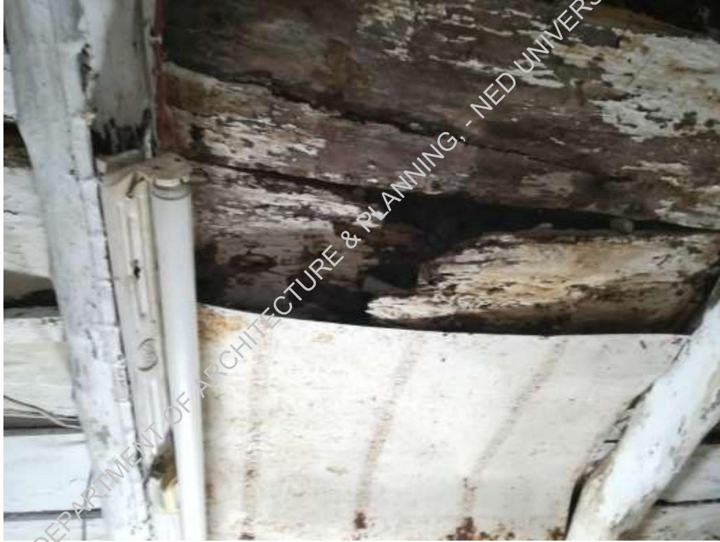
Plate-4: timber slab in bad condition,
