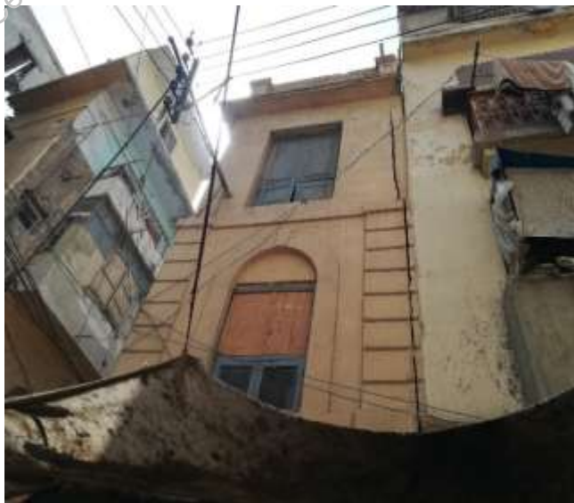
Plate-2: Vertical separation cracks at the right-side façade of building observed at rear side
