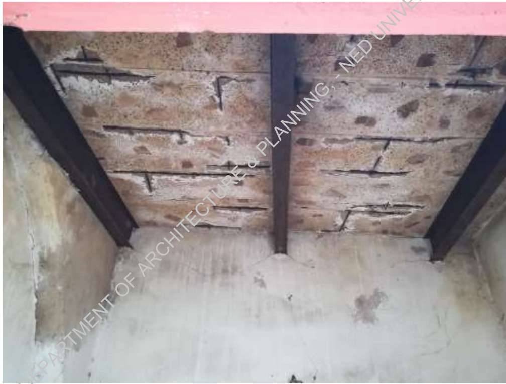
Plate-6: Concrete construction done later on, in bad condition
