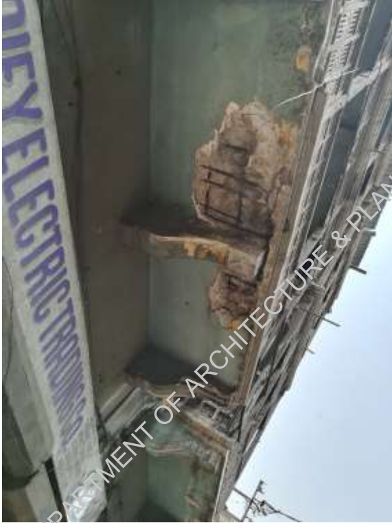
Plate-6: reinforcement of original projections exposed
