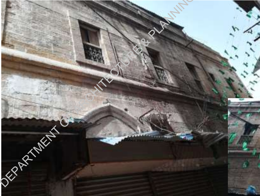
Plate-1: Front Façade- loose stone masonry can be noted at places. Additional floor on top is also visible
