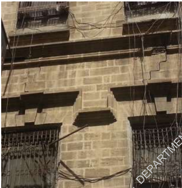
Plate-2: Wide cracks at façade
