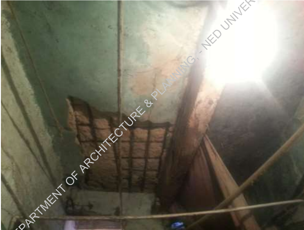
Plate-8: RCC construction deteriorating
