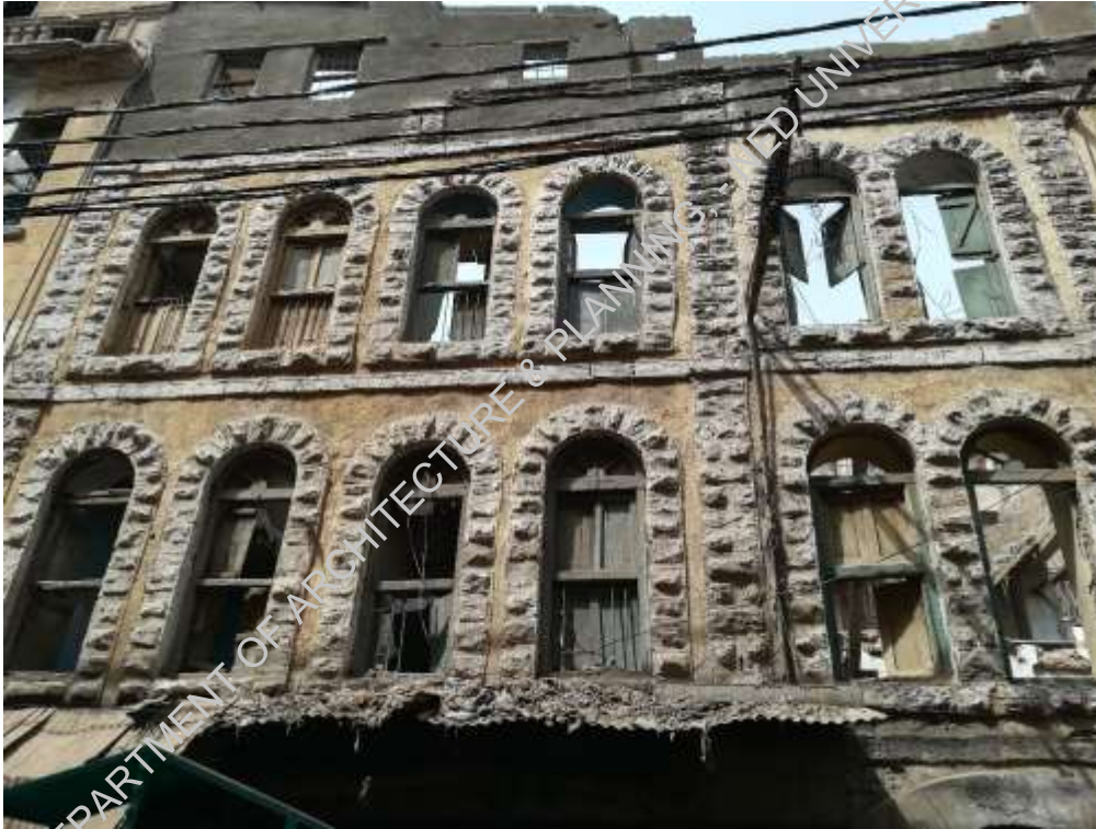
Plate-8: masonry at rare façade in bad condition
