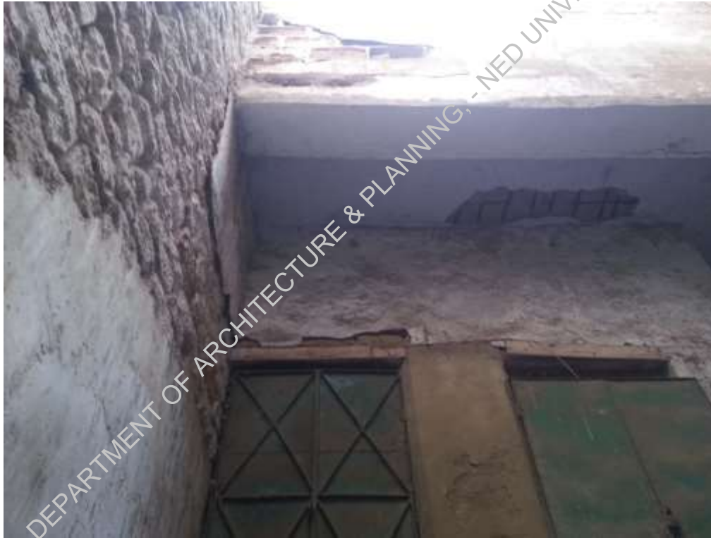
Plate-6: Loose stone masonry is visible
