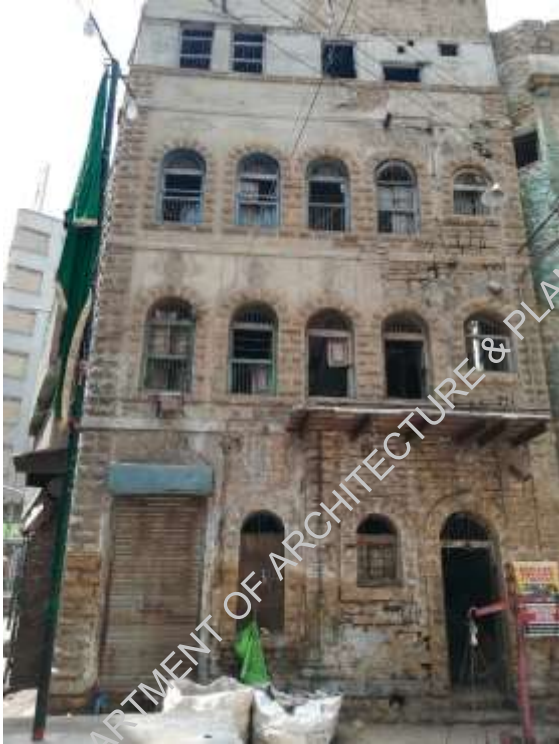
Plate-1: Front Façade- loose stone masonry can be noted at many places. Additional floor on top is also visible
