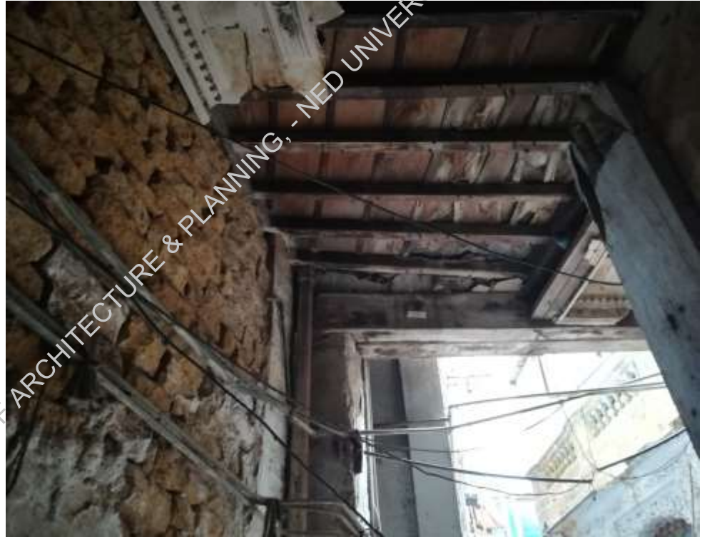
Plate-4: Timber slab in bad condition.
