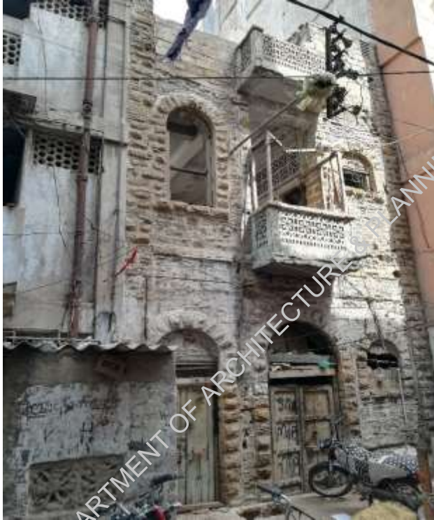
Plate-1: Front Façade- loose stone masonry can be noted at many places. Additional floor on top is also visible
