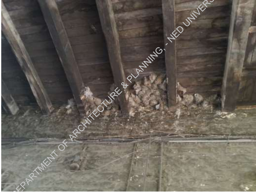
Plate-6: Termite infestation near main entrance.
