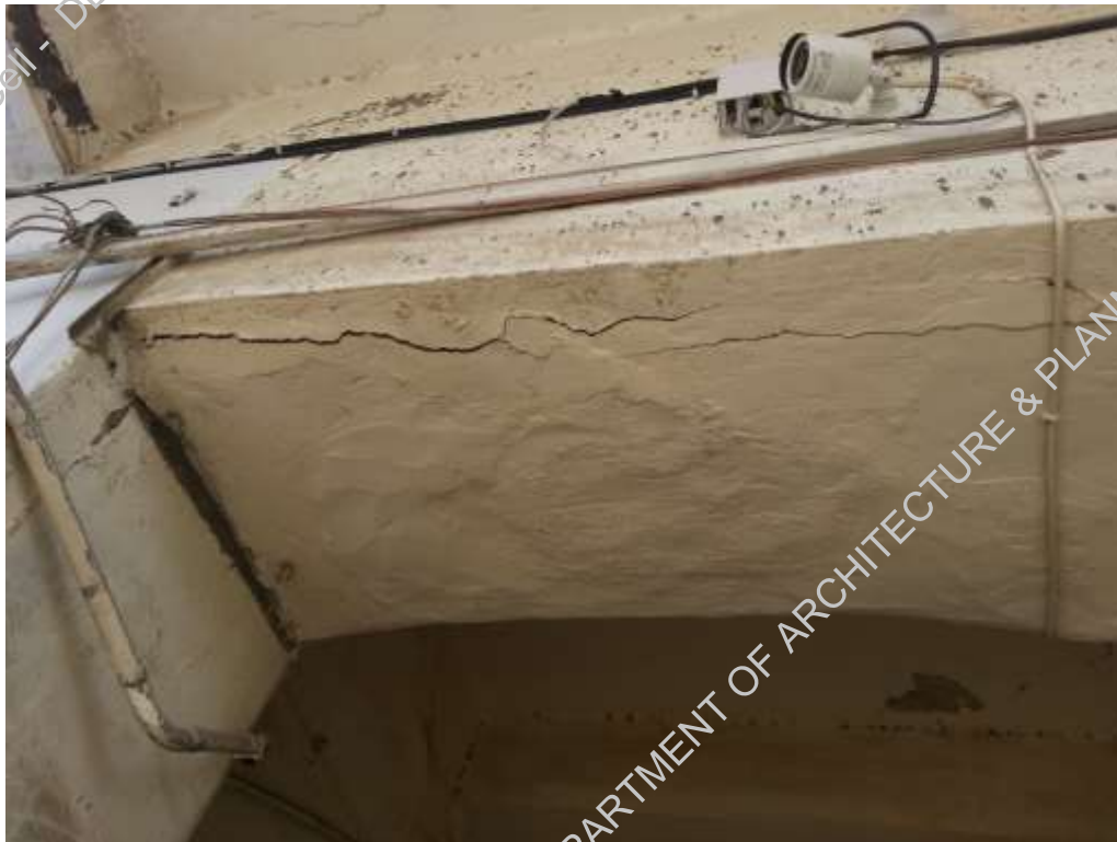
Plate-9: Bad condition of Beam above stair
