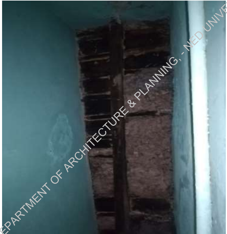
Plate-7: Bad condition of roof slab due to seepage.
