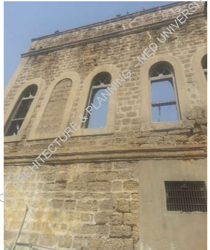
Plate-3: mortar has been eroded
