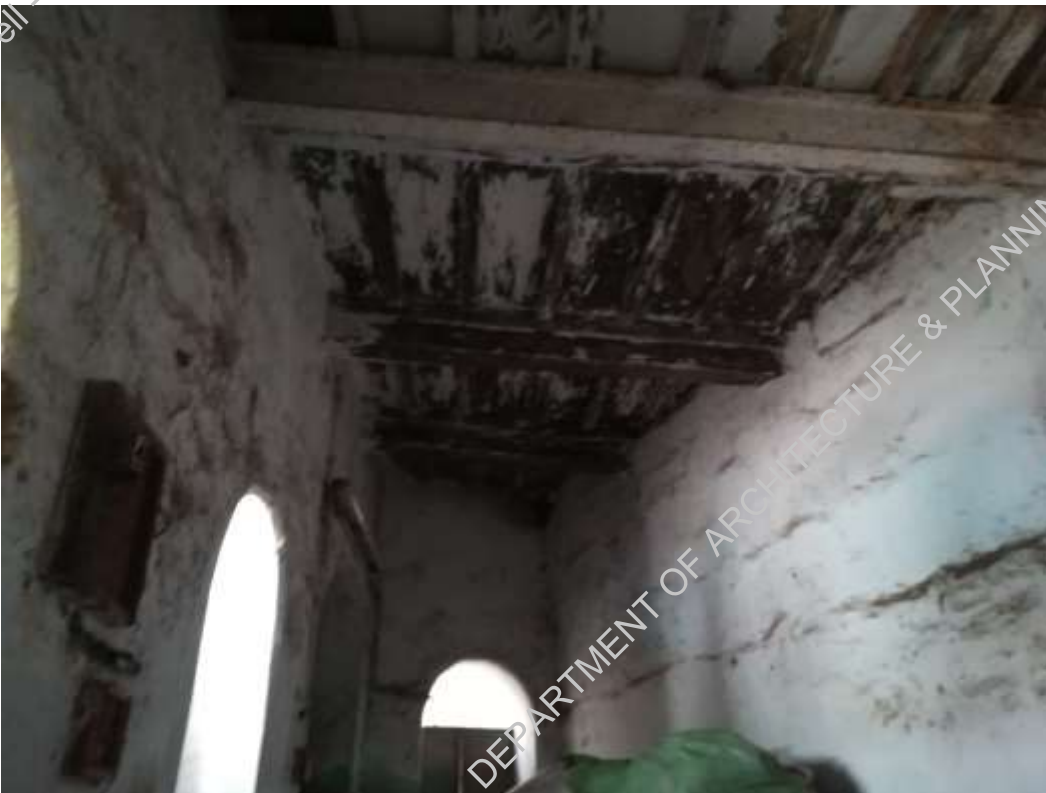
Plate-5: steel girders installed to support existing slab
