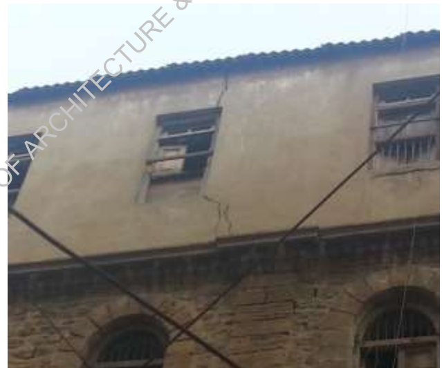
Plate-3: crack in wall of intervention at roof
