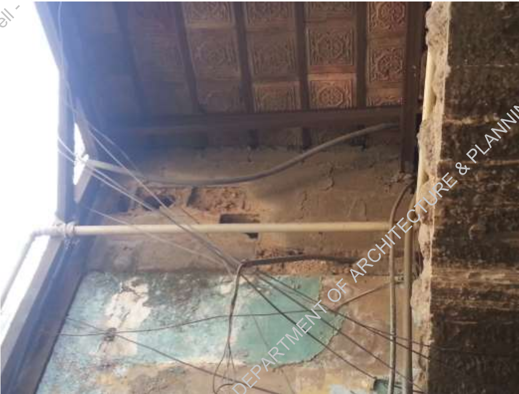
Plate-7: Stone masonry being punctured for various reasons
