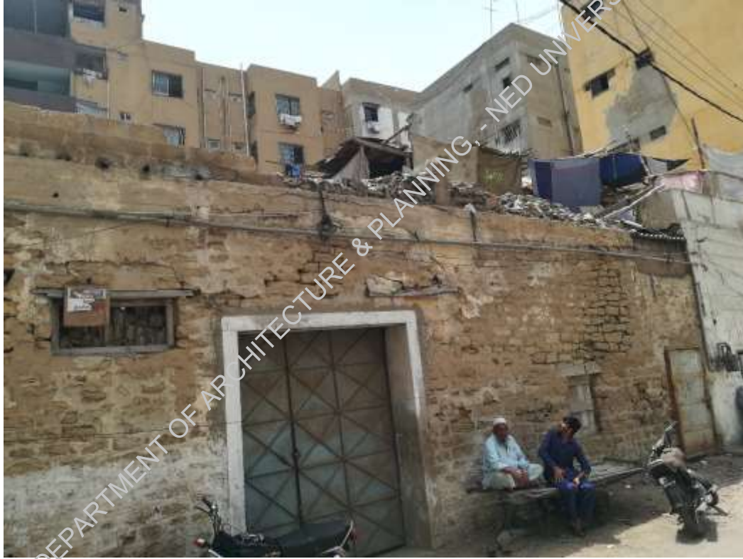
Plate-4: Loose stone masonry is visible
