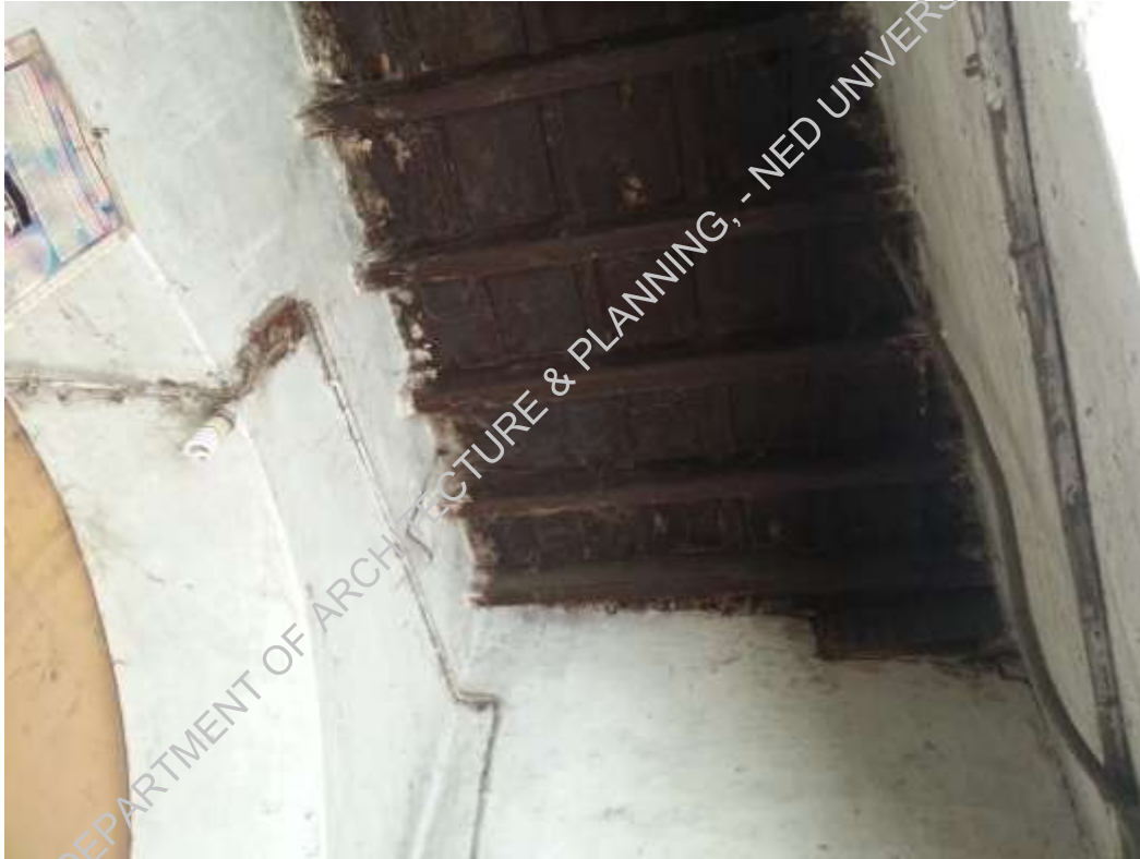
Plate-4: timber slab is in good condition,
