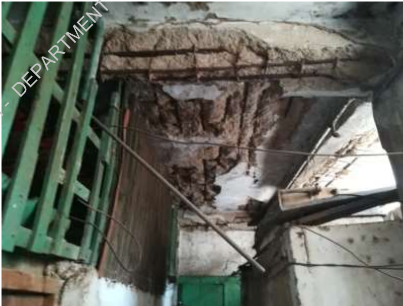
Plate-9: Bad condition of reinforced concrete construction of central court
