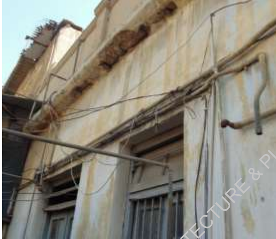
Plate-6: slab projection in bad condition
