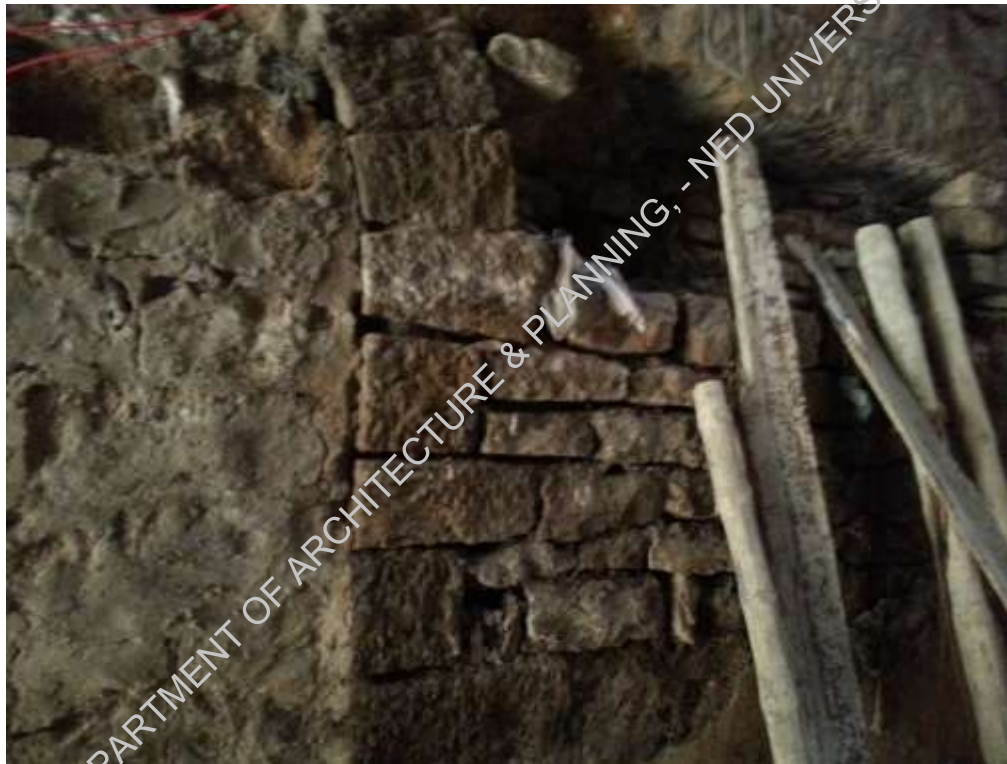
Plate-6: Loose stone masonry is visible
