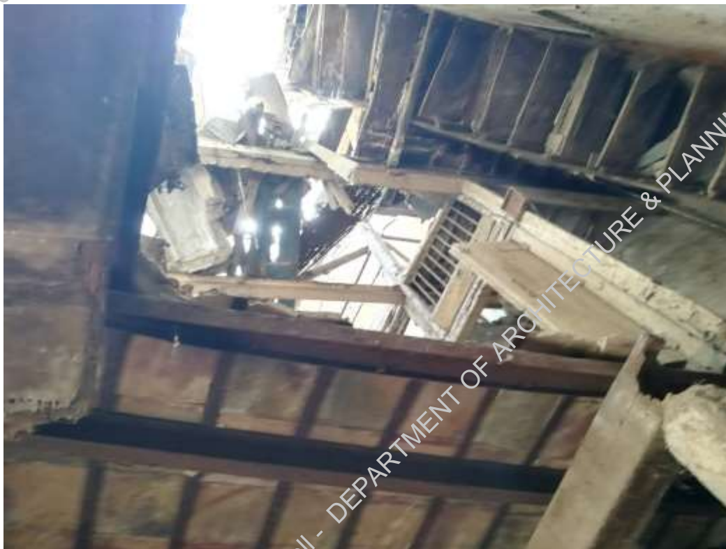
Plate-7: slab and stair collapsed
