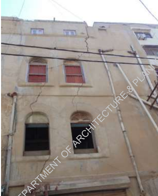
Plate-2: Wide cracks at the rear façade of building before collapse
