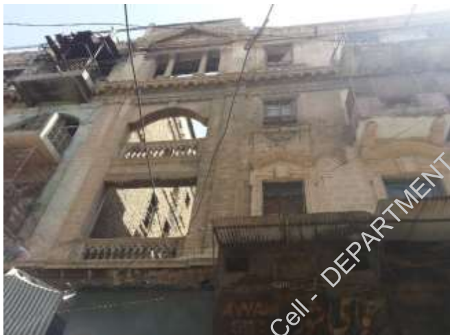
Plate-2: Wide cracks at the rear façade of building before collapse
