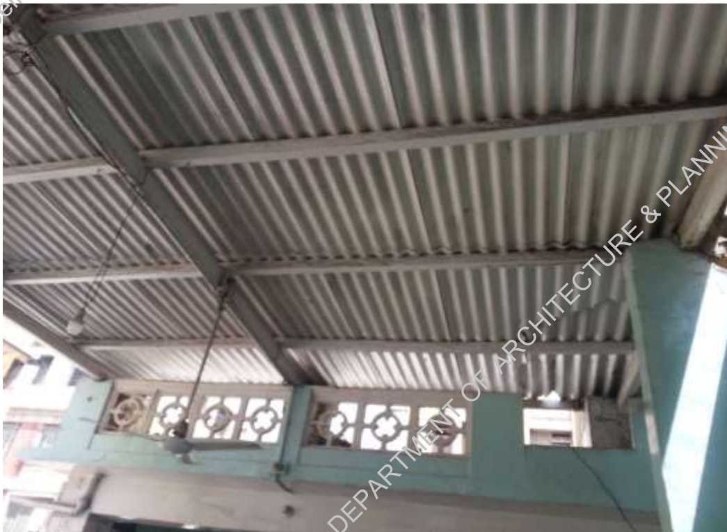
Plate-4: Temporary roof above
