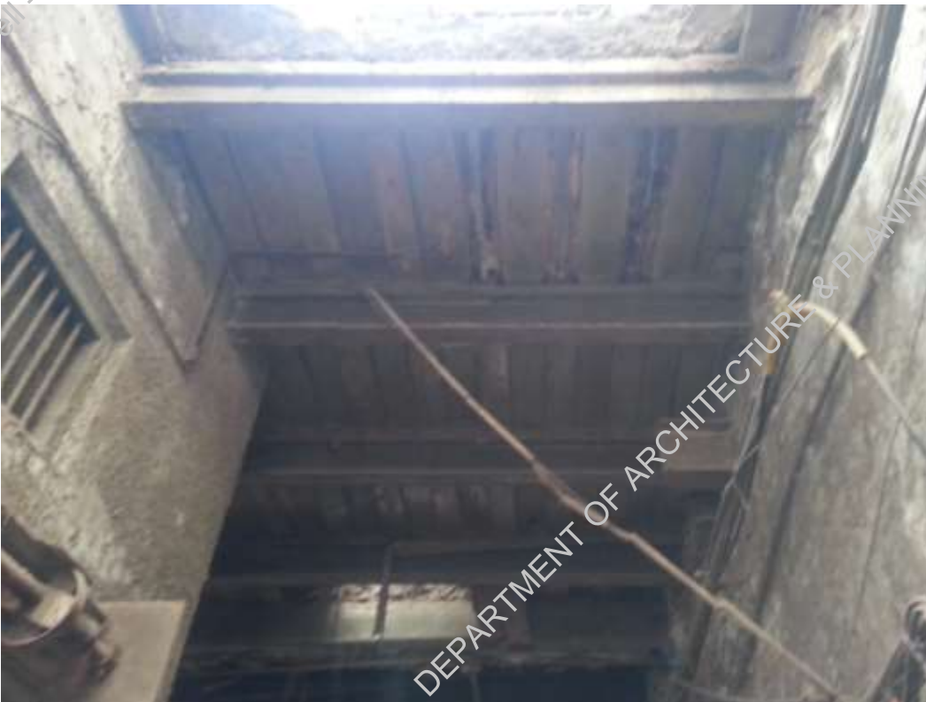
Plate-5: slab crumbling
