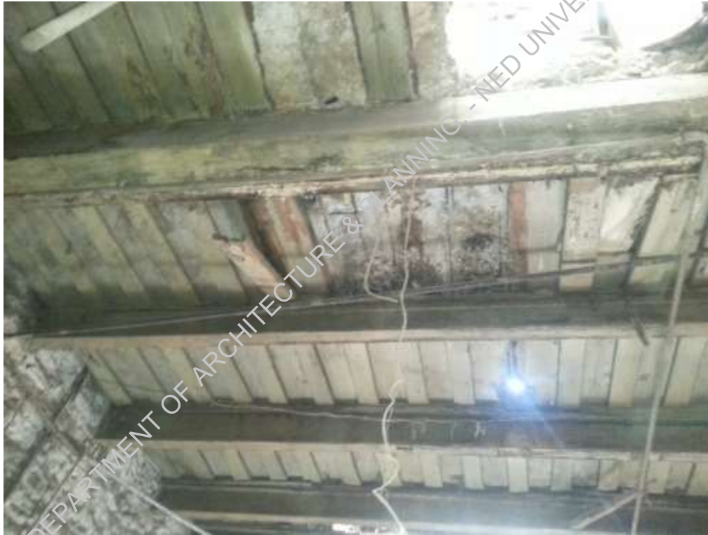
Plate-6: Bad condition of original timber flooring and walls at ground floor
