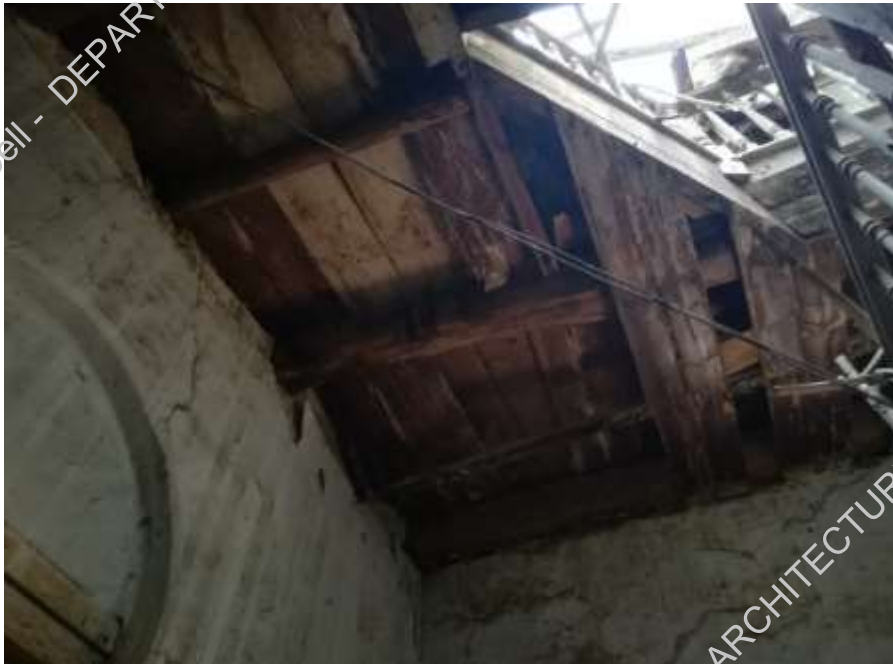
Plate-6: Loose planks
