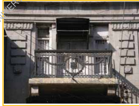
Centre balcony on second floor
