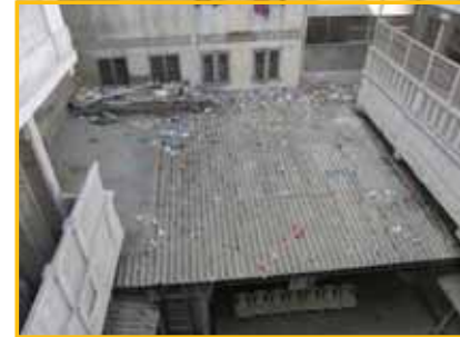
Asbestos shed over waiting area
