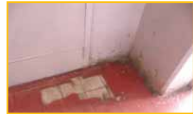
Tiled floor underneath Vinyl tiles
