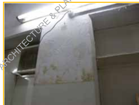
Internal wall Paint
