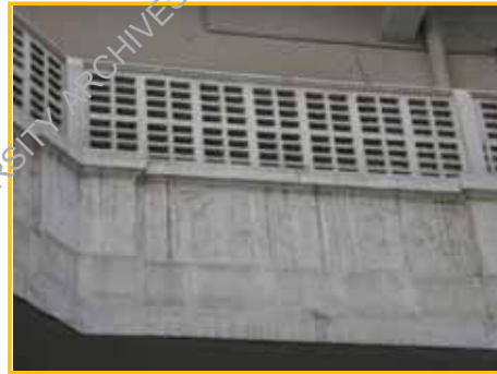
Altered interior parapet which still have traces of original design
