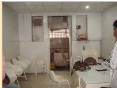
Alteration of windows and ventilators of Hakim Said's room
