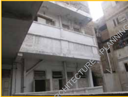
Toilet blocks of first floor
