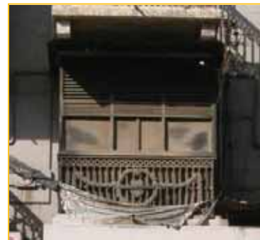
Balcony of first floor
