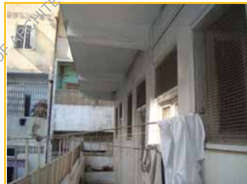
Installation of net, replacing timber windows of hall on second floor
