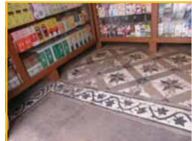
Original flooring at shop
