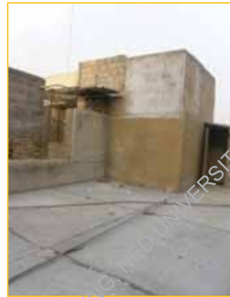
Exposed drainage lines, water tank of adjacent building is also seen
