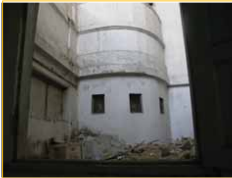
View of the duct area from first floor
