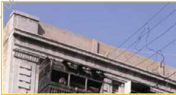
Replaced parapet wall
