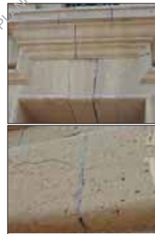
Figure 85 (a, b). Mortar Cracks filled with Cement Mortar
