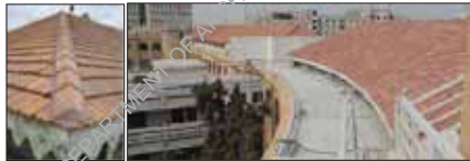
Figure 29 (a, b, c). Pitched Roof Covered with Khapraail Tiles
