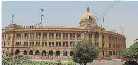
Figure 1. Front View of KPT Building facing M. A Jinnah Road
