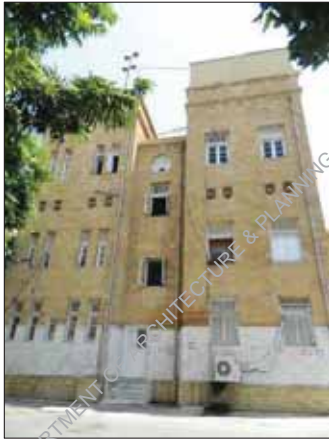
Figure 41. Exposed Plumbing Services on Building's rare side
