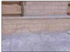
Figure 61. Moisture Stains
