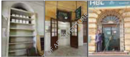
Figure 47 (a, b, c). Altered Doors
