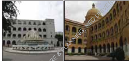
Figure 36(a, b). Addition of monument, asphalt pavement & hedges along building
