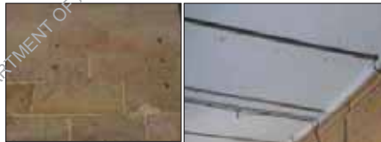
Figure 68 (a, b). Iron Nails on Stone Walls and Ceiling of Corridor
