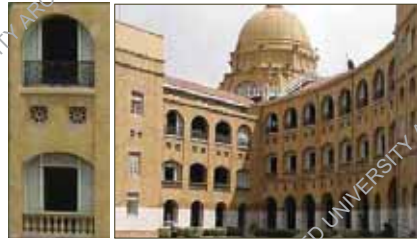
Figure 18. Arch Openings Figure 19. Building rare size facing courtyard
