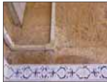
Figure 51. Staining of Stone
