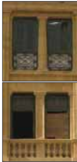
Figure 21 (a, b). Twin Windows of 1 st & 2 nd Floor
