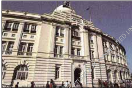
Figure 37. KPT Building Coated With an Off White Paint Coat
