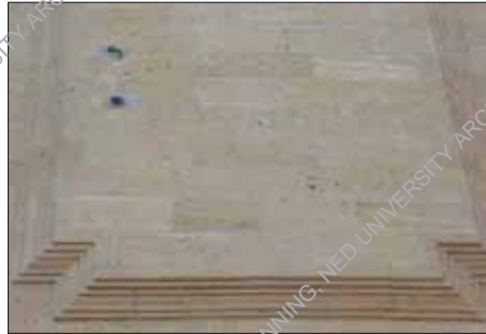
Figure 71. Cement Mortar Grouting in Holes Drilled for Some Installations
