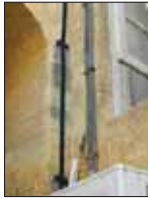
Figure 69. Ferrous anchors stain
