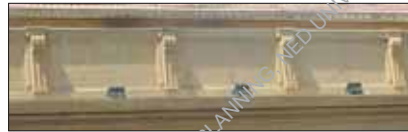
Figure 30. Brackets under the Edge of Pitched Roof
