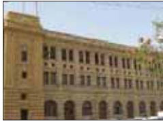
Figure 33. Custom House Building
