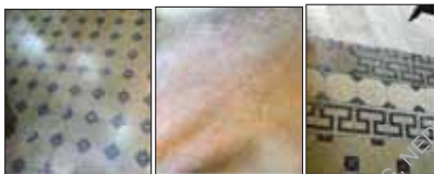
Figure 31 (a, b, c). Pigmented CC Flooring
