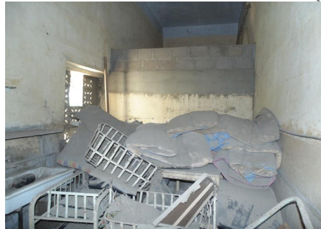
Figure -36 Partition Wall at Backside Corridor
