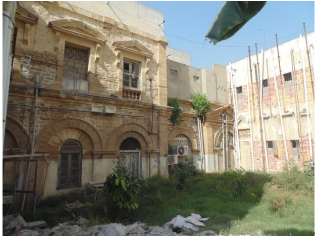
Figure-26 Extension Blocking Side Façade
