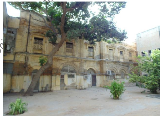
Figure-30 Openings Closed with Masonry
