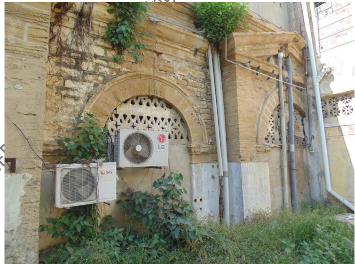
Figure-44 Micro Biological Growths at the Rear Side of OPD
