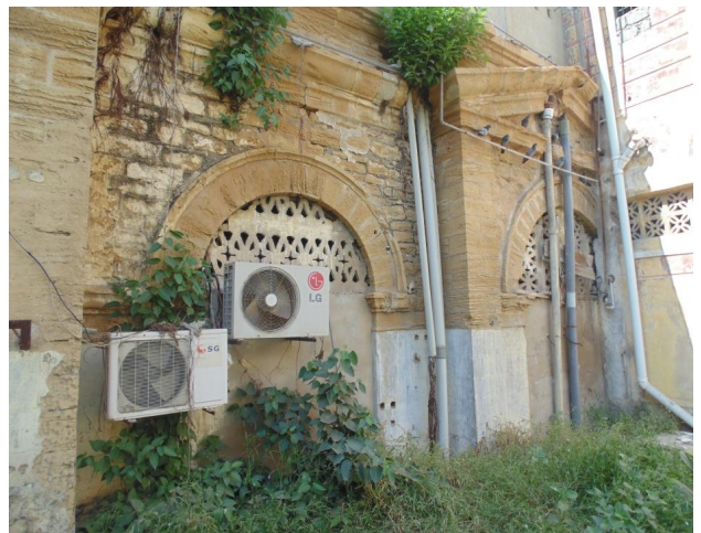
Figure-48 Micro Biological Growths at the Rear Side
