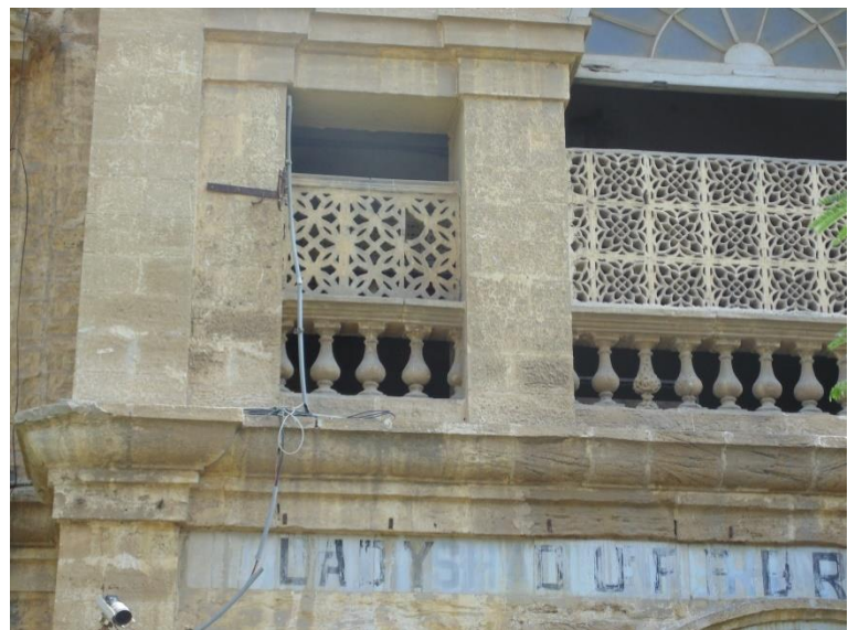
Figure-34 Iron Nails on Front Façade
