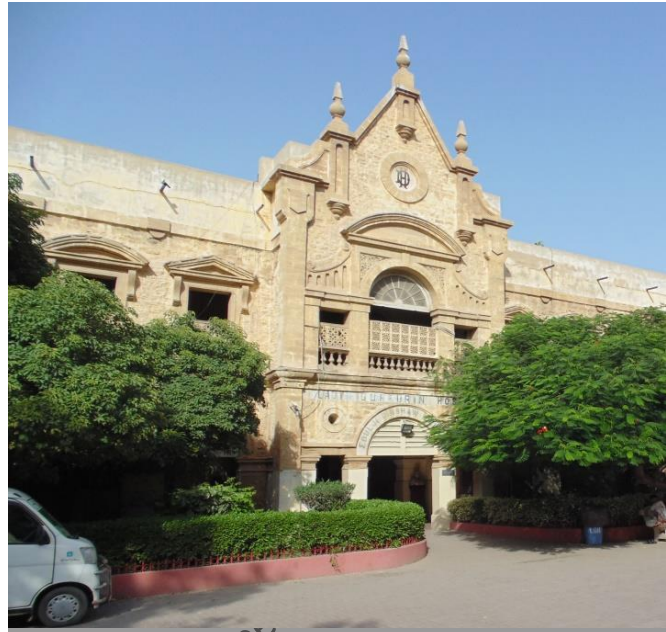
Figure-11 Central Entrance of the Building
