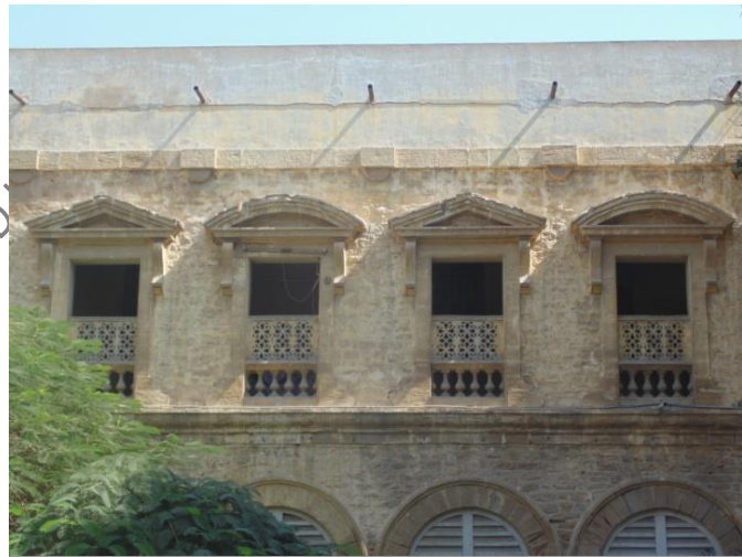
Figure-12 Use of C.C. Jalis on at Front Façade
