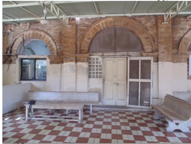
Figure-24 Covered Waiting Area at OPD Women Section
