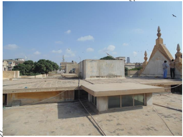
Figure-27 Gable Roof replaced with Flat Roof
