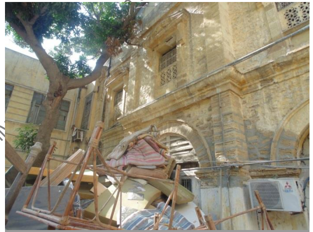
Figure-47 Mortar Joints Filled with Cement Plaster on Rear Façade
