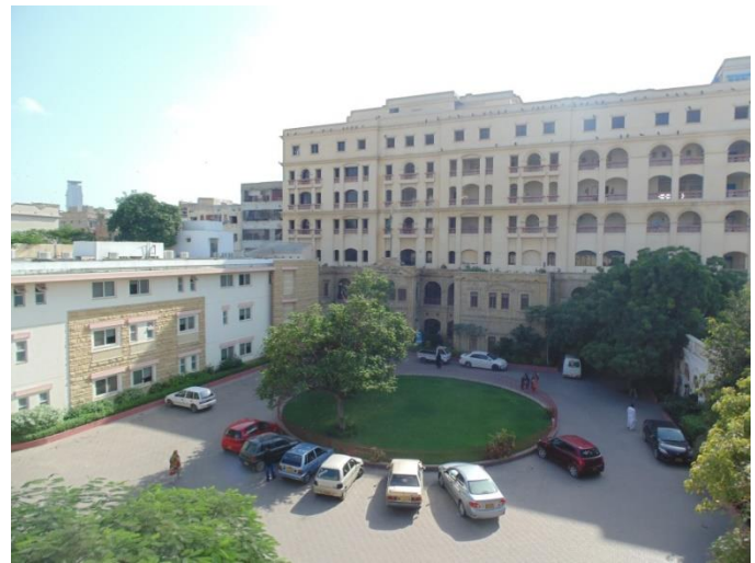
Figure-5 Central Hub of Site
