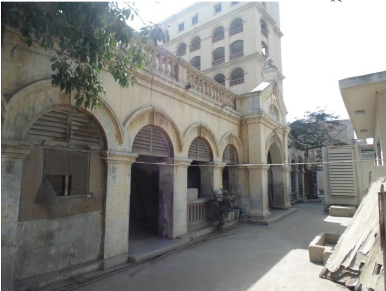
Figure-3 Stone Structure (Isardas Asonmal Dispensary)
