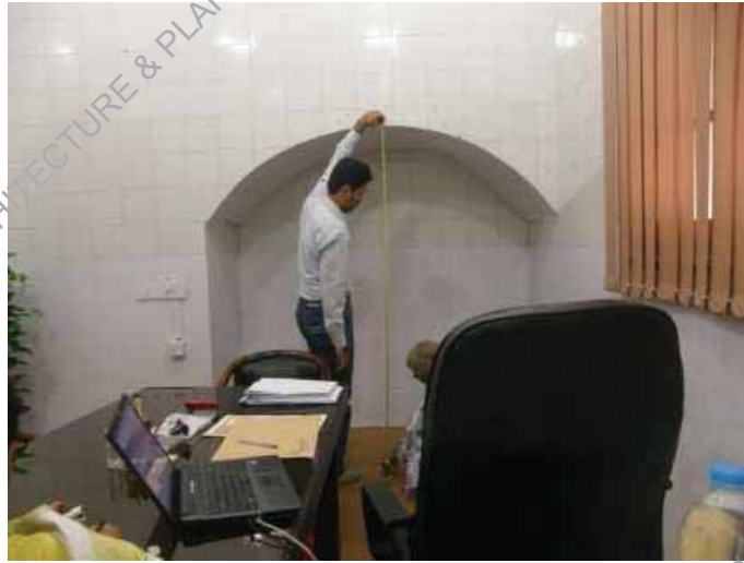
Kitchen converted into an office where the original chimney is sealed from inside.
