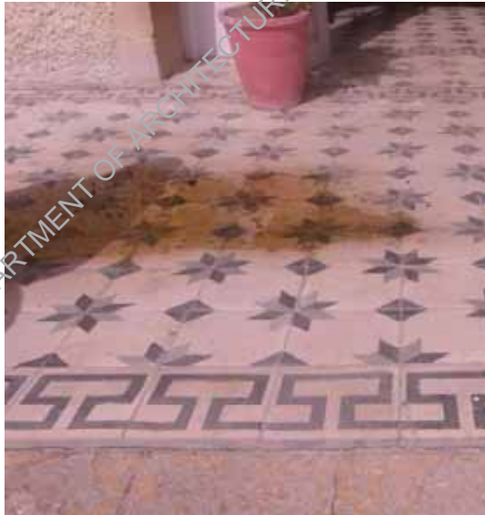
Pictures showing faulty slopes in flooring of patio located on western side, causes frequent presence of water on it.
