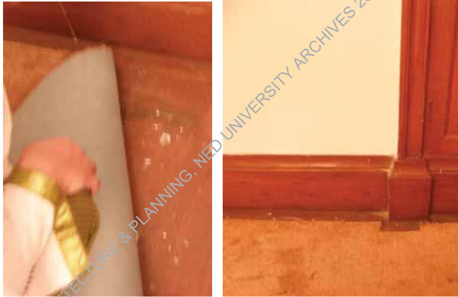
The wooden flooring and skirting in conference room on ground floor, showing stains of carpet adhesive.
