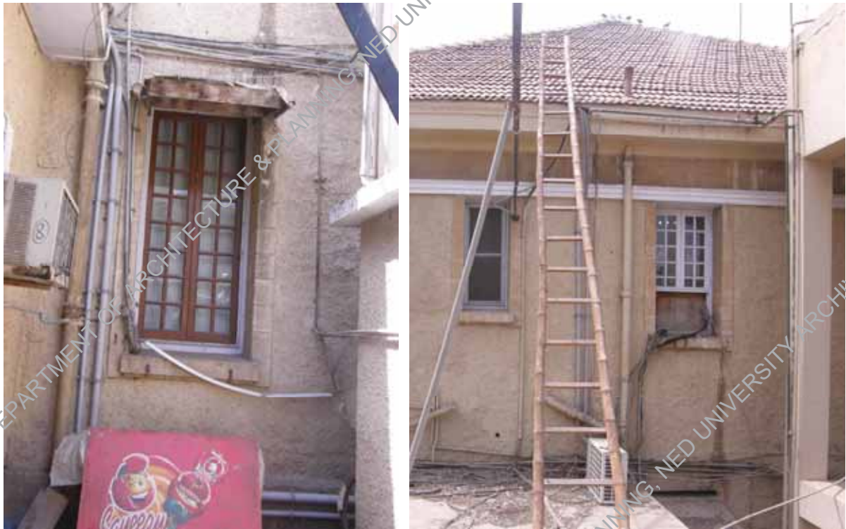
Different views of northern façade showing haphazardly installed electrical wiring and plumbing pipe.
