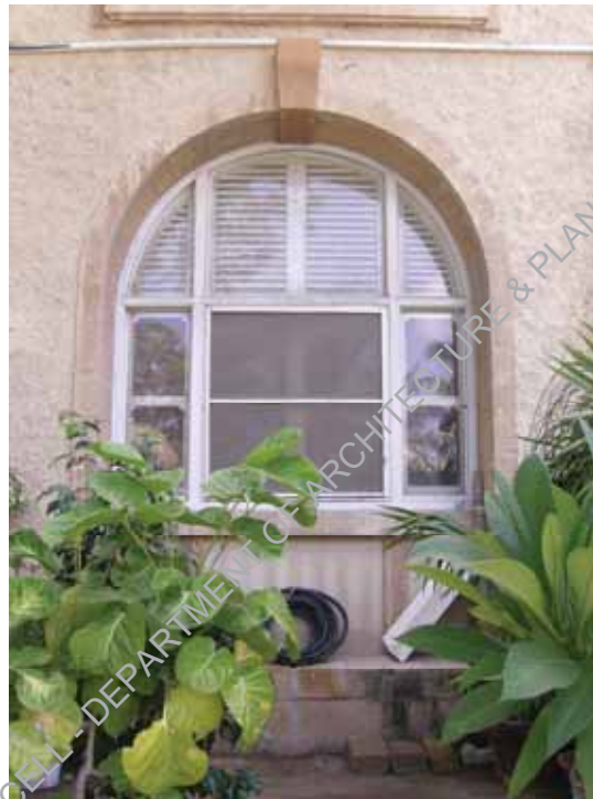
The window on western side of the building is being altered by filling the parapet with cement mortar and by adding the net frames.
