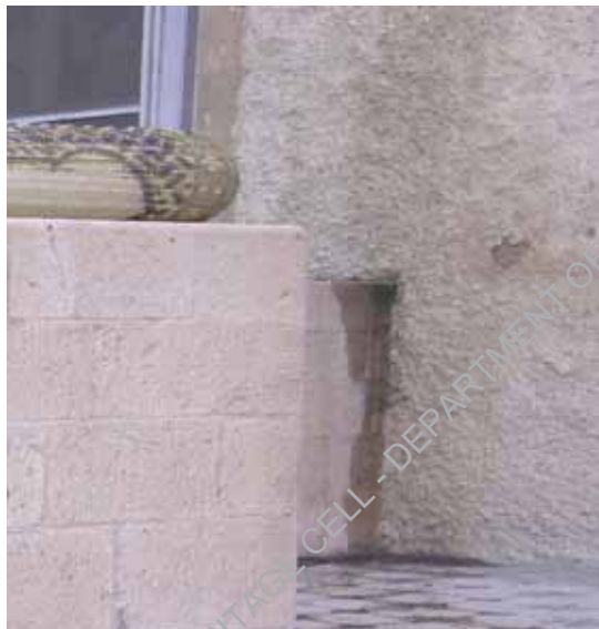
Seepage and moisture stains due to localized water sources.
