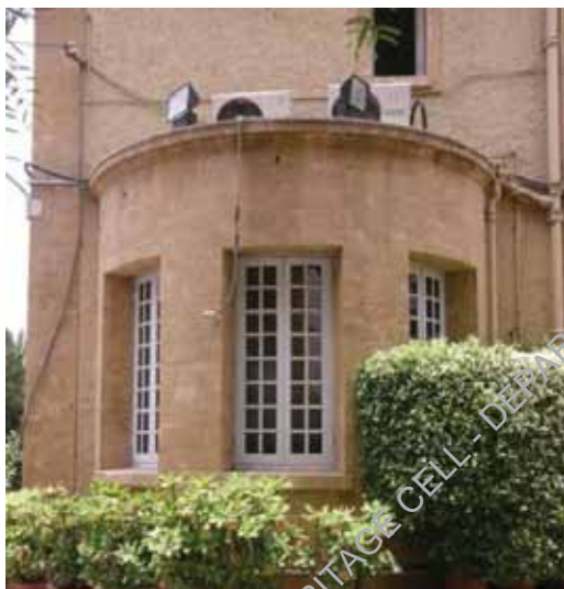
Semi circular niche on ground floor showing the original dressed stone masonry.
