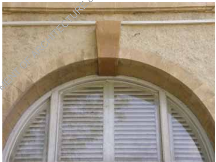
External surfaces covered with dana plaster
