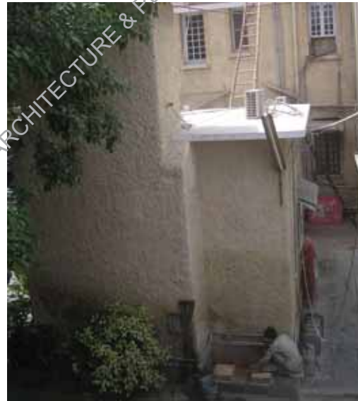
Seepage and moisture stains due to localized water sources.
