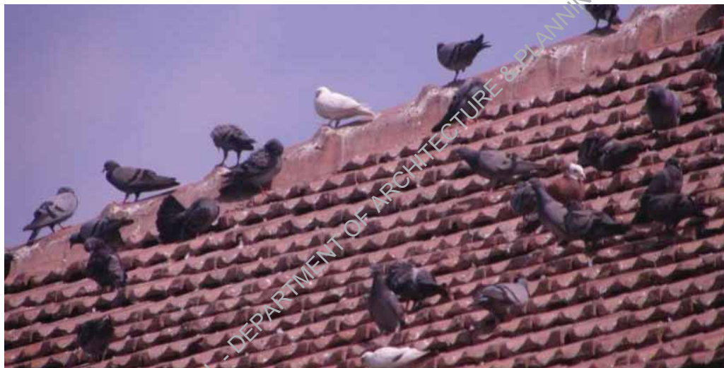
Red khuprail tiles, showing stains of bird's droppings.
