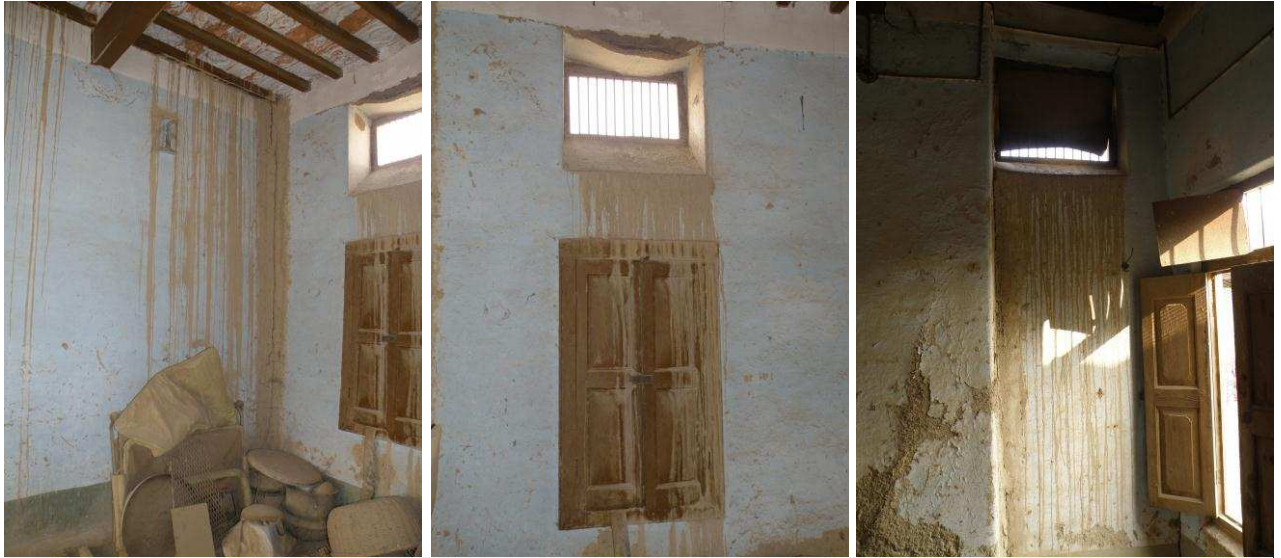
Images showing water coming from windows/ ventilators
