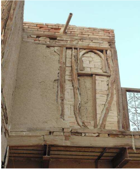
Brick masonry construction having timber reinforcements.
