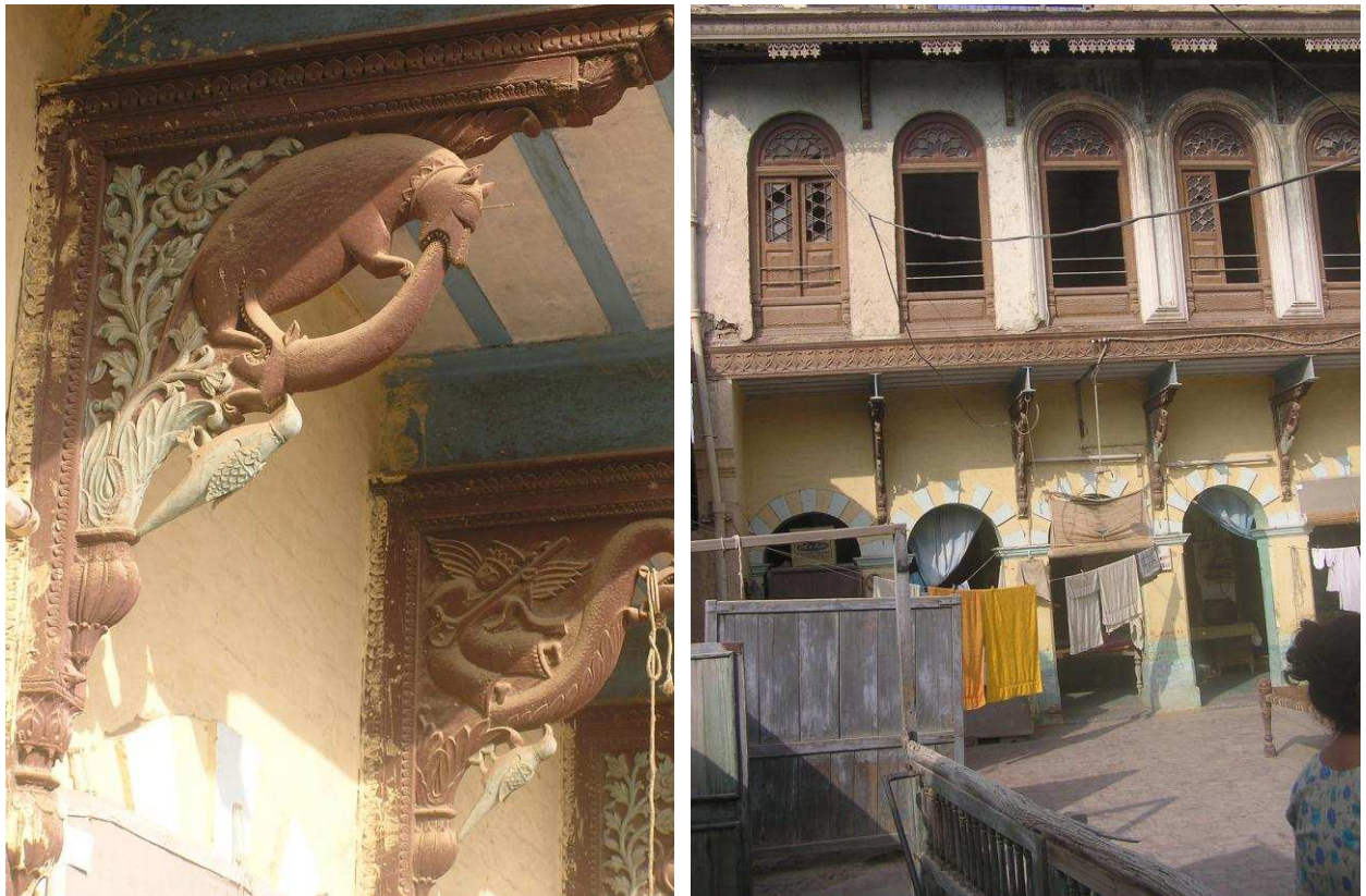
Carved timber brackets supporting upper floor cantilever (left). Courtyard facing façade (right).
