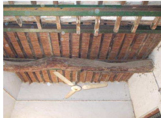
Ceiling of a room - combination of original and new roof.
