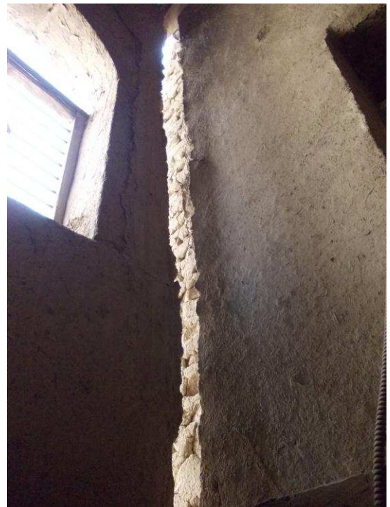
Detached masonry wall causing a deep vertical opening.
