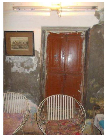
Damage caused by rising dampness.
