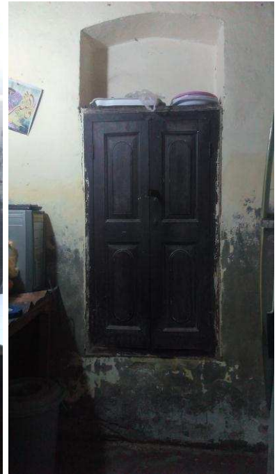
Visible signs of rising dampness on ground floor walls
