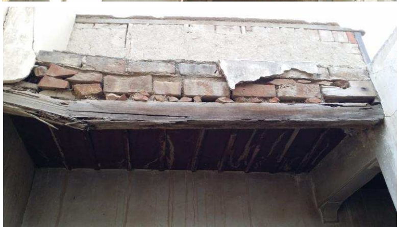
Sagging of ceiling and floor due to broken beams and timber planks.
