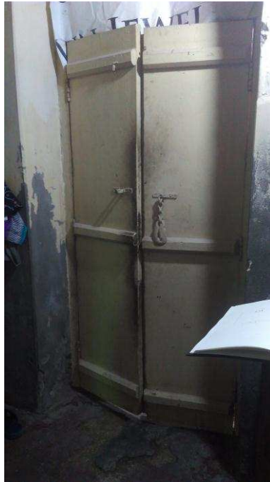
Visible signs of rising dampness on ground floor walls
