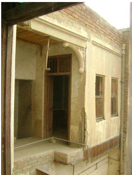
Detachment of plaster and loss of bonding between wall and plaster
