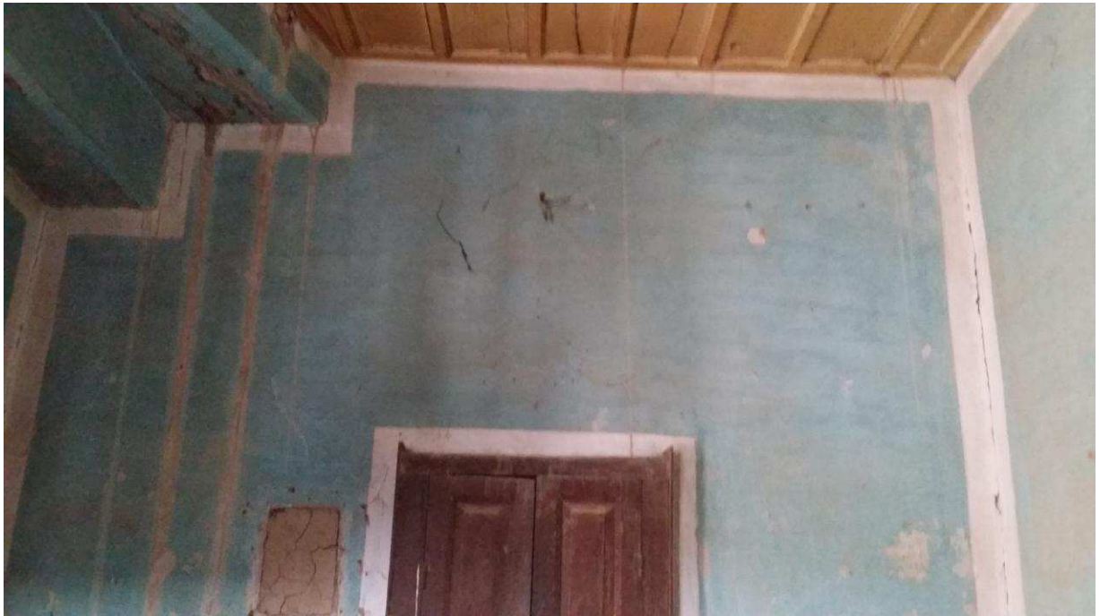
Rain water penetration from roof is evident from dripping water stains on the walls
