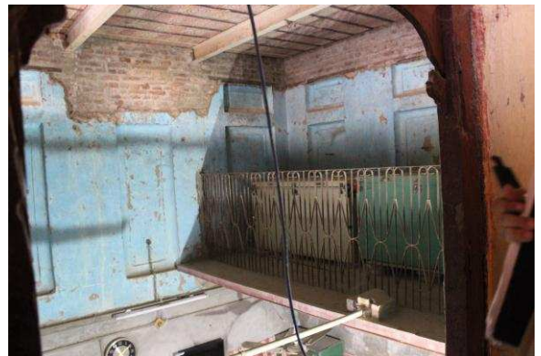
Damaged wall plasters
