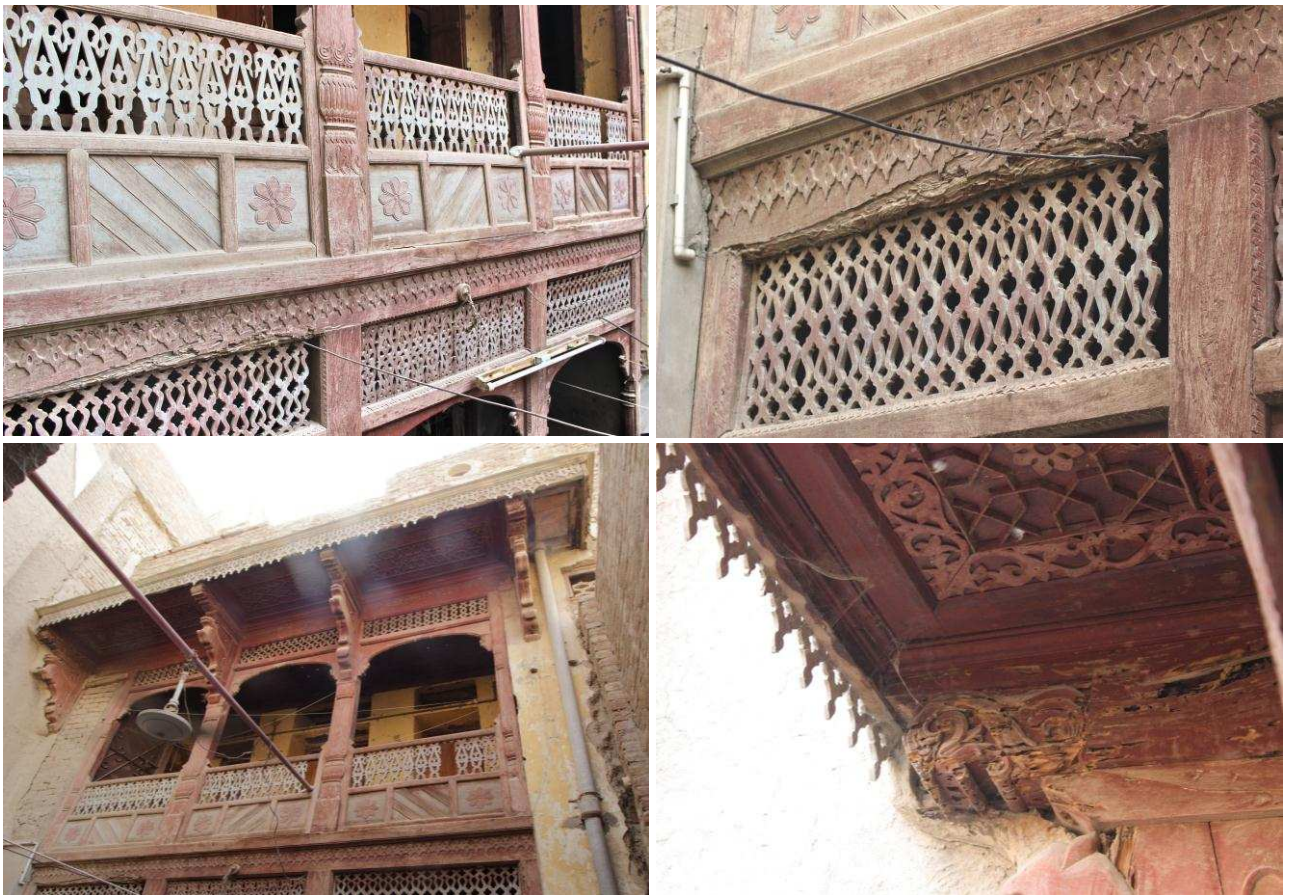
Various areas showing signs of decaying woodwork.
