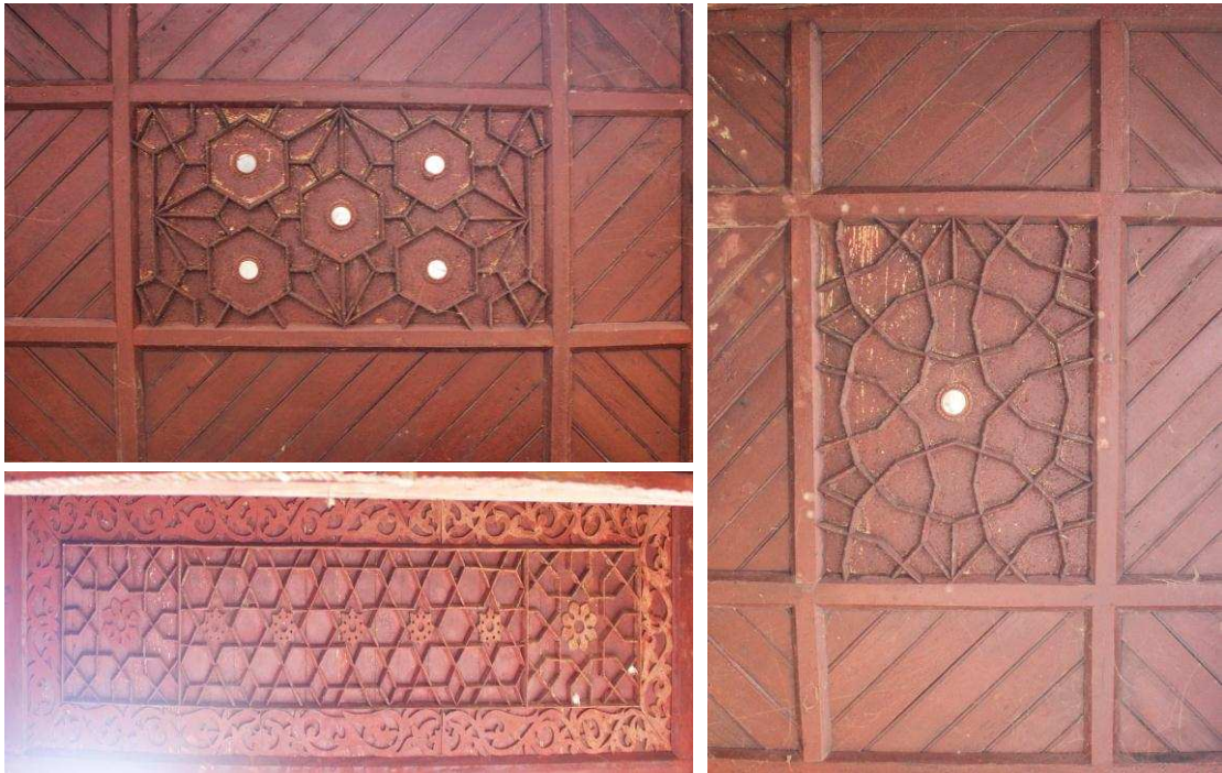
Detail of qab-sazi work on ceilings.
