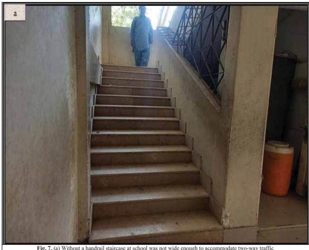
Fig. 7. (a) Without a handrail staircase at school was not wide enough to accommodate two-way traffic
