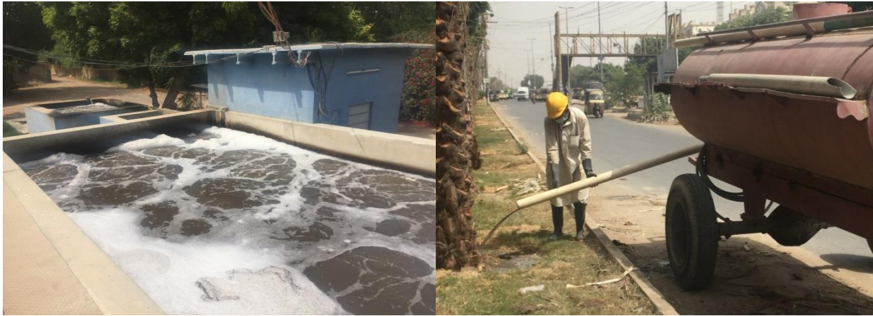
Wastewater aerobic treatment and use for plant watering
